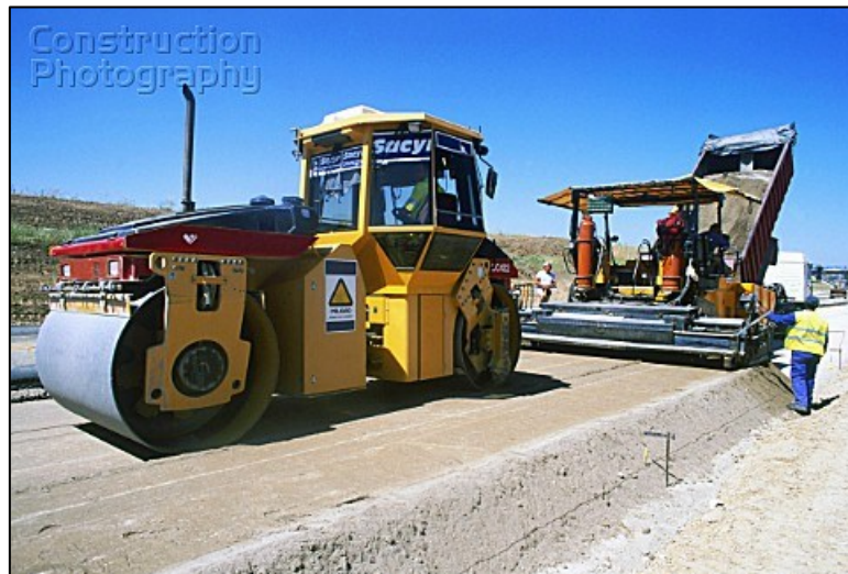
Figure 8: Aggregate Laying.
