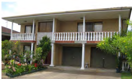
Figure 1: Front façade (Case 1) (Source: Authors)
