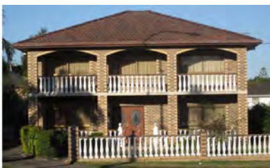
Figure 10: Front façade (case 4) (Source: Authors)
