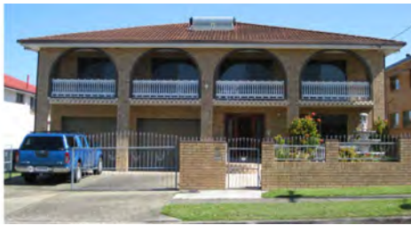
Figure 7: Front façade (case 3) (Source: Authors)
