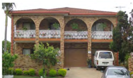
Figure 4: Front façade (case 2) (Source: Authors)
