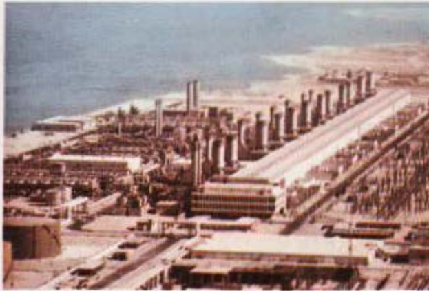
Fig. 1: A View of Ras Abu Fontas Power and Water Station (Adapted from reference (2)).
