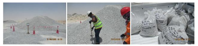
Fig. 2: RCA material stockpile and sampling at QPMC
