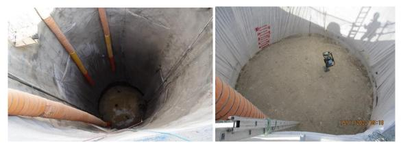
Fig. 1: Temporary shafts on the WWDNB project used for micro tunneling and manhole installation (left side) and ongoing conventional backfilling works (right side)
