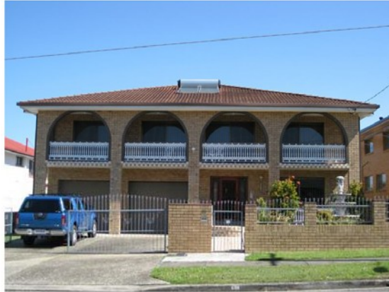
Figure 18. The main facade. House built in 1983 by Flavia and Aldo. The main facade is characterized by a steel balustrade, brick columns supporting the concrete slab on the front porch and arches on the balcony. (Photo by the author)
