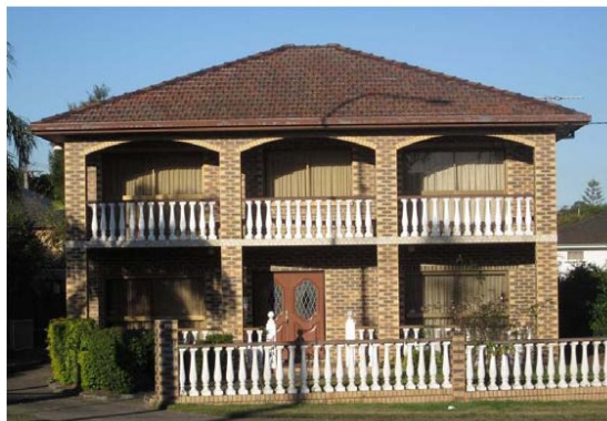
Figure 24. The main facade. Case 4: House built in 1984 by Pina and Carmelo. The main facade is characterized by a hand made concrete balustrade and brick columns supporting the concrete slab on the front porch and elliptical arches on the balcony. (Photo by the author)
