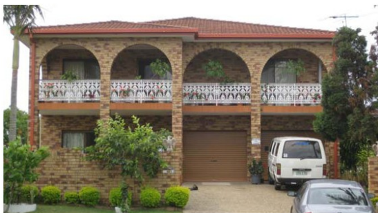
Figure 12. The main façade. House built in 1982 by Maria and Salvatore. The main façade is characterized by a steel balustrade, brick columns supporting the concrete slab on the front porch and arches on the balcony (Photo by the author)
