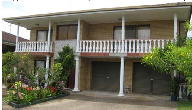
Figure 1. The main façade. The house was built in 1983 by Lina and Vittorio. The main façade is characterized by a hand made Concrete balustrade and Roman columns supporting the concrete slab on the front porch (photo by the author)
