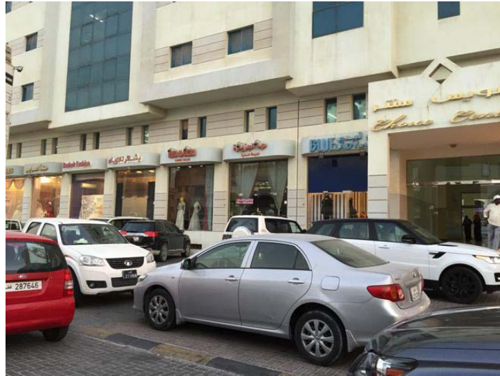
Figure 11. Inadequate Parking Locations
