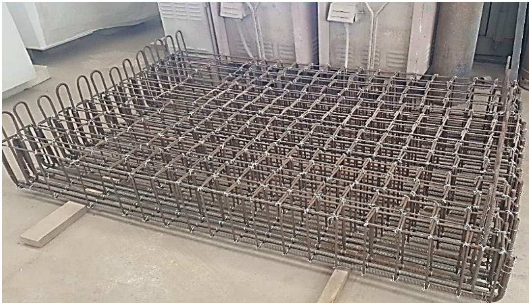
Figure 22: Steel cages preparation.
