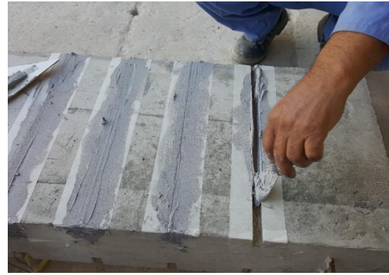
(b) Fill the \frac{1}{2} of the groove by epoxy
