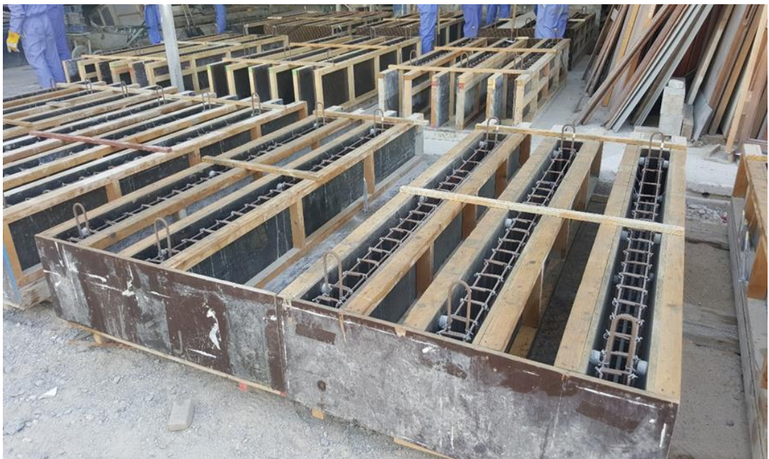
Figure 24: A wood framework for beam specimens.
