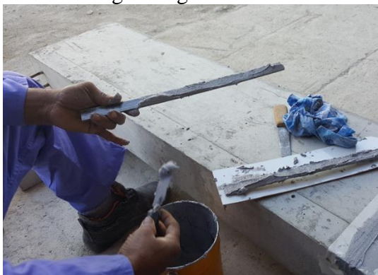
(c) Cover FRP strips by epoxy
