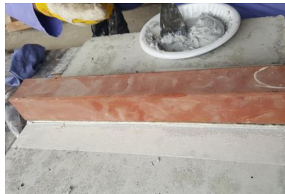
(f) Place a weight to fix the FRP in place
