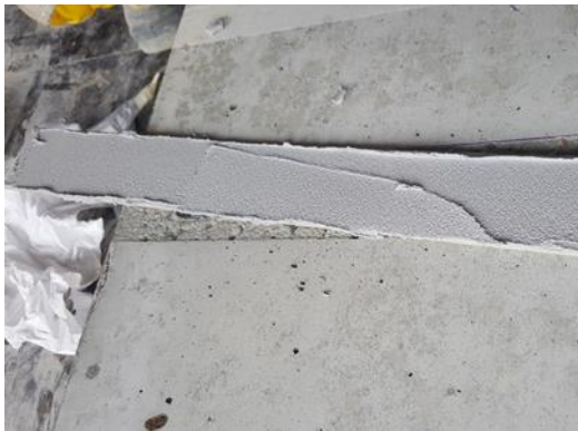
(c) A layer of epoxy on the FRP strip
