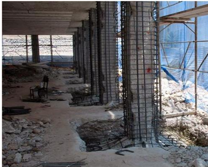
Figure 2: RC columns were jacketing [41].
