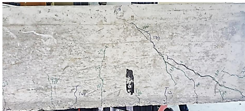
Figure 38: Crack pattern and failure mode for reference specimen, R-S0.
