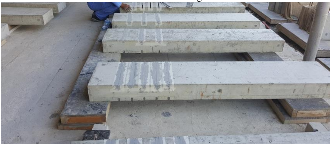
(e) The final shape of the beam specimens after NSM strengthening from one side.
