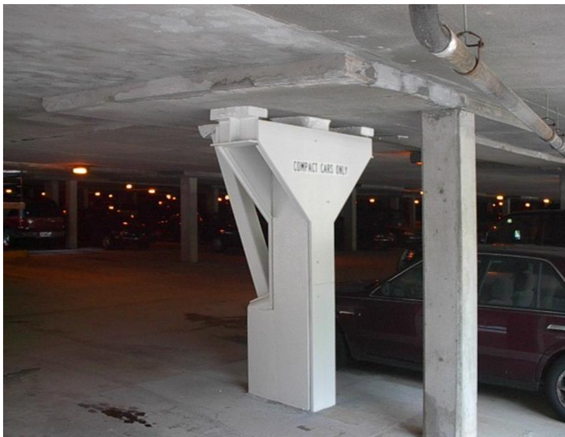
Figure 5: Strengthening of parking garage slab by span shortening [44].
