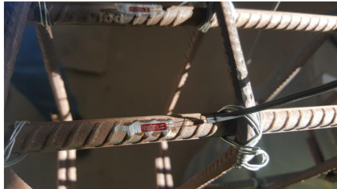
(a) Installation the strain gauge on the prepared surface in the flexure bars
