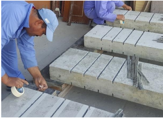
(a) Prepare the beam for strengthening
