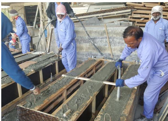
(c) Vibrating the concrete to avoid unwanted air voids
