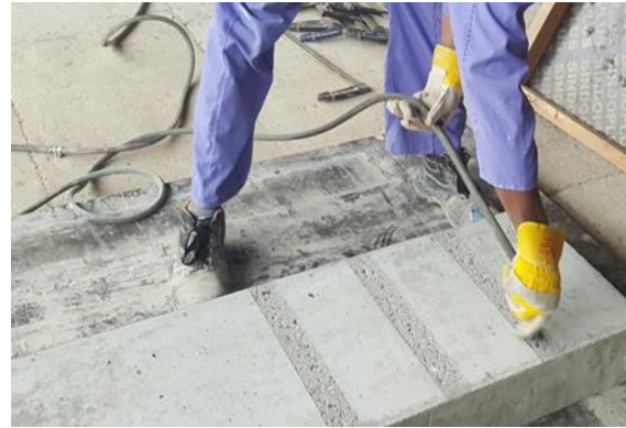
(b) Clean the surface by compressed air
