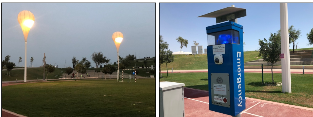
Figure 75. Lightings and emergency device in Oxygen Park
