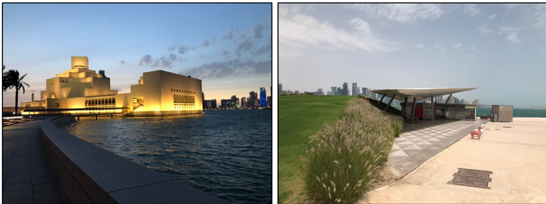
Figure 29. The type of buildings within the MIA Park boundary
