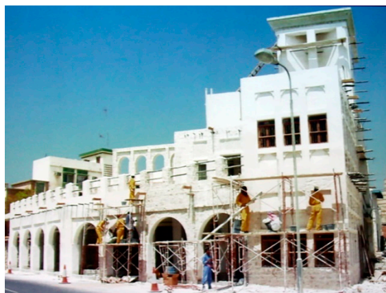
Figure 14. The use of non-local, non-traditional materials on existing traditional vernacular buildings (restoration or reconstruction: a dilemma).
