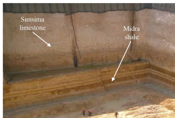
Figure 1: Vertical cut showing the subsurface stratification at one of construction sites in Doha
