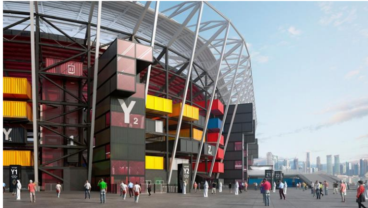
Figure 8. Modular design of Ras Abu Aboud stadium
