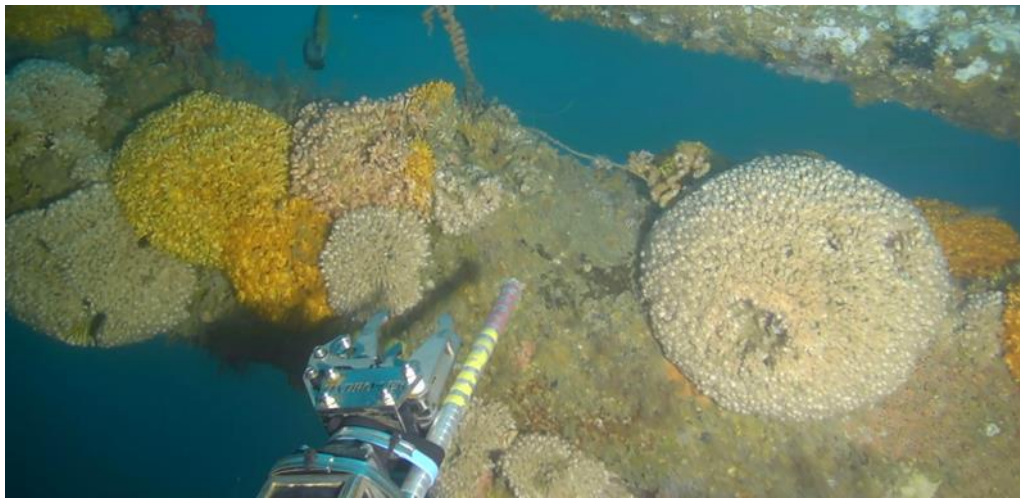
Figure 4. ROV while surveying AL-Shaheen platforms
