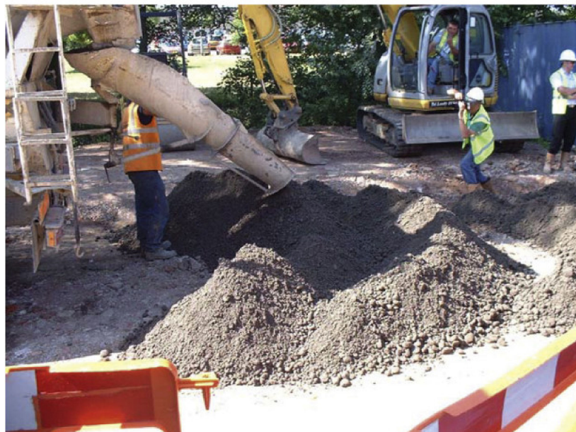
Figure 2. Semidry concrete for a road foundation. Reproduced from [52].
