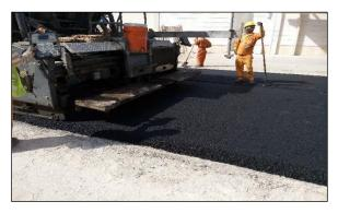
Fig. 3: Paving Operations of Asphalt Mix with 15% RAP
