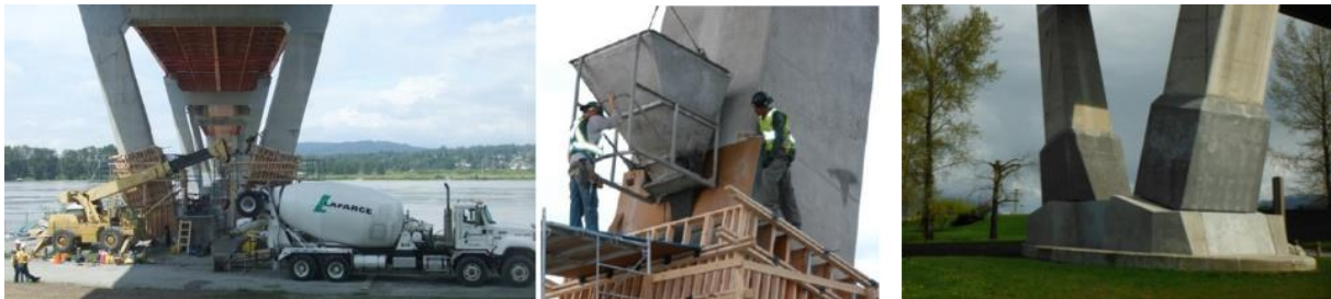
Fig. 3: Mission Bridge Seismic Retrofit Project Abbotsford, British Columbia, Canada, Doiron (2016)
