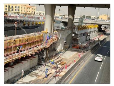
Fig. 9: – Median Piers during construction
