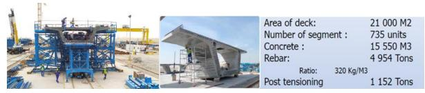
Fig. 4: Precast Concrete Segment Fabrication in VSL Yard 50 kms. south of Doha
