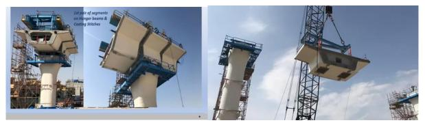
Fig. 5: Precast Concrete Segment Installation for Junction B6 bridge
