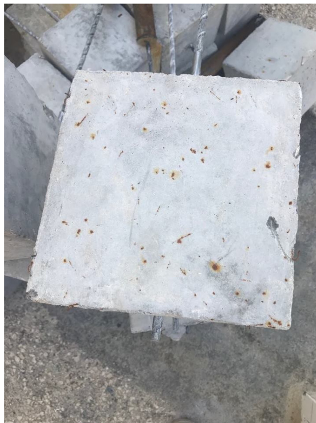
Fig. 11. Corrosion of Steel Fibers in SFRC.
