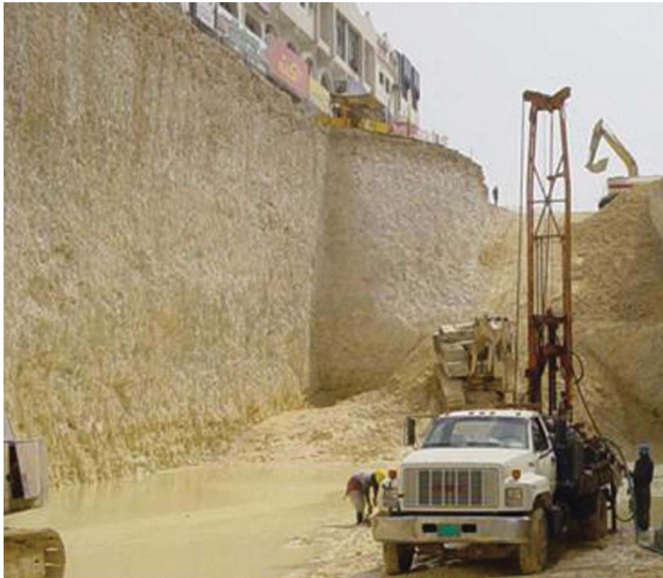
Fig. 3. Vertical cut that shows a typical extent of limestone layer in this study area.
