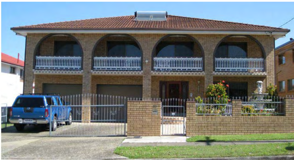
Figure 8 (Case 3). House built in 1983 by Flavia and Aldo. The main façade is characterized by a steel balustrade, brick columns supporting the concrete slab on the front porch and round arches on the balcony (photo by the author, 2012)
