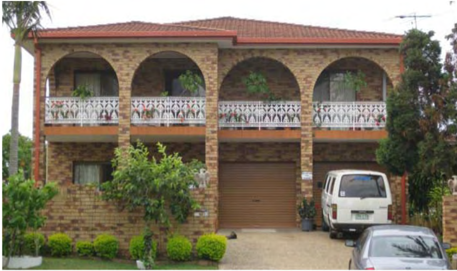
Figure 7 (Case 2). House built in 1982 by Maria and Salvatore. The main façade is characterized by a steel balustrade, brick columns supporting the concrete slab on the front porch and round arches on the balcony (photo by the author, 2012)
