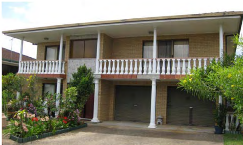
Figure 6 (Case 1). The house was built by Lina and Vittorio. The main façade is characterized by a hand made concrete balustrade and Roman columns supporting the concrete slab on the front porch (photo by the author, 2012)
