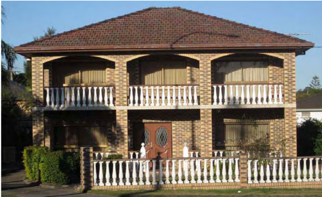
Figure 9 (Case 4). House built in 1984 by Pina and Carmelo. The main façade is characterized by a hand made concrete balustrade and brick columns supporting the concrete slab on the front porch and elliptical arches on the balcony (photo by the author, 2012)
