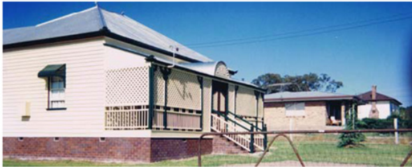
Figure 18. Renovated house. In 1967 Pasquale and Assunta purchased a weatherboard house standing on timber stumps in Bracken Ridge. In 1972 the renovation of the house was completed. A brick basement wall around the perimeter of the house replaced the original timber stumps. The external weatherboard walls were sanded and painted to maintain the original look of the house. (Photo from case 14)
