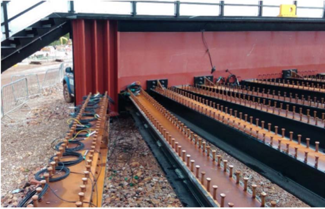
Figure 1. Installation of fibre-optic sensors on a bridge
