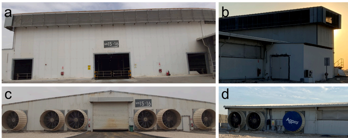
Fig. 3. Pictures of barn B: (a) inlet end, (b) inlet end side view, (c) exhaust end, and (d) exhaust end side view.
