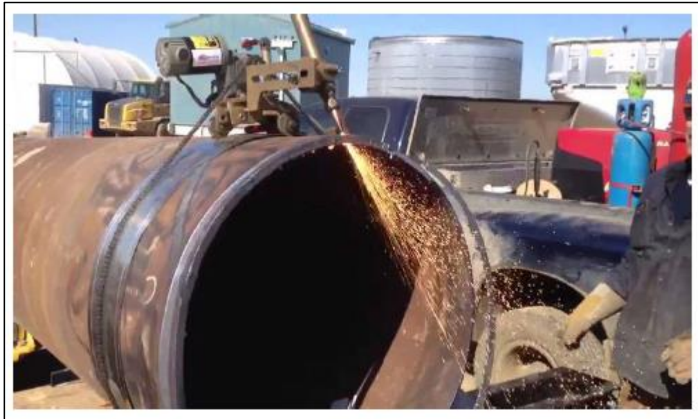
Figure 11. Pipe bevelling
