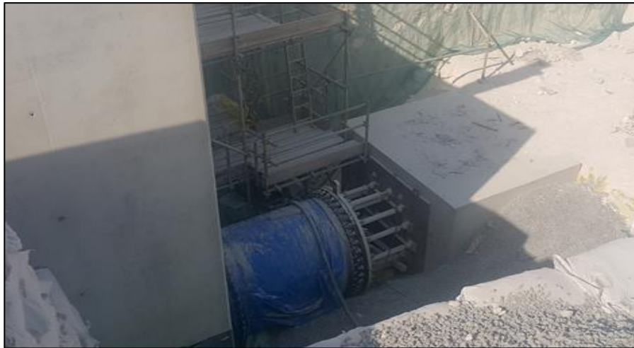
Figure 15. Hydro-testing activity
