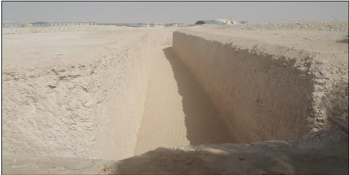
Figure 8. Trench preparation "U-shape & pipe bedding."
