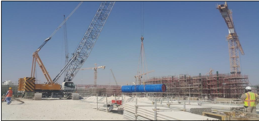
Figure 9. Shifting pipes inside the trench
