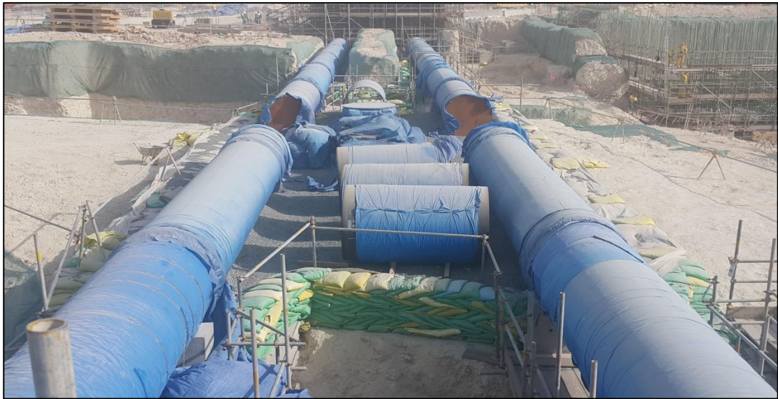
Figure 10. Fit-up and stringing in the trench
