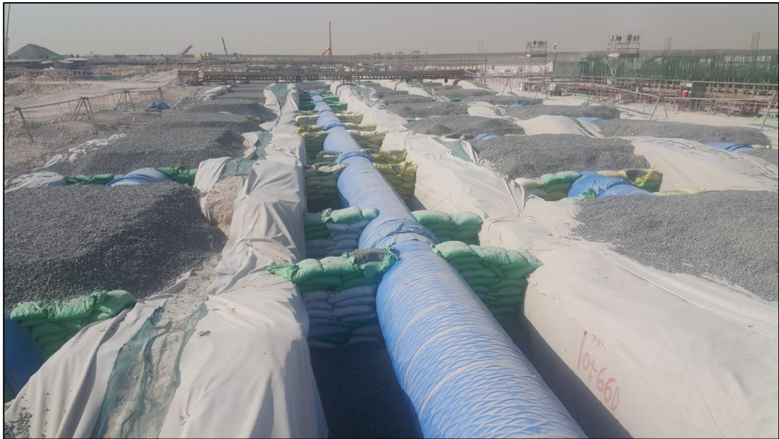
Figure 14. Partial backfilling
