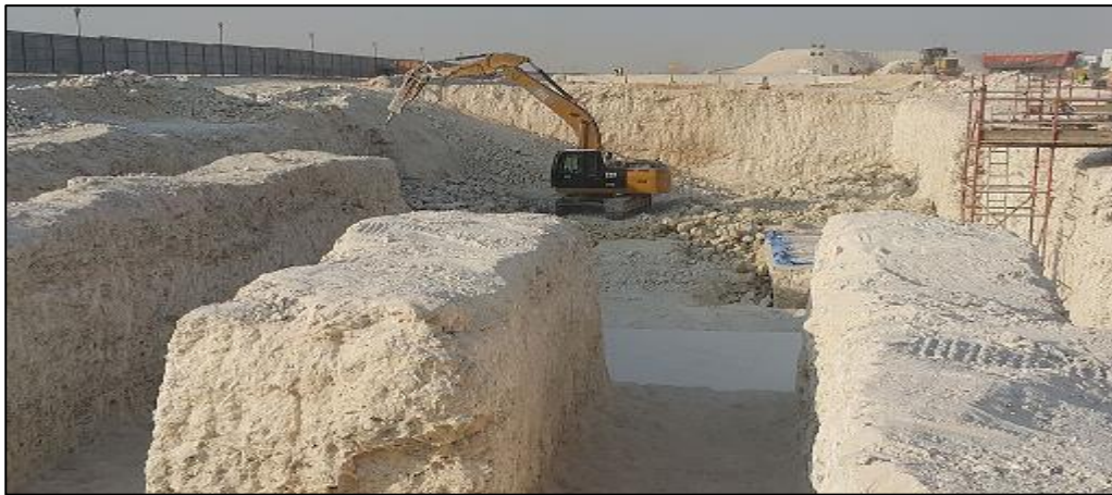
Figure 7. Trench excavation
