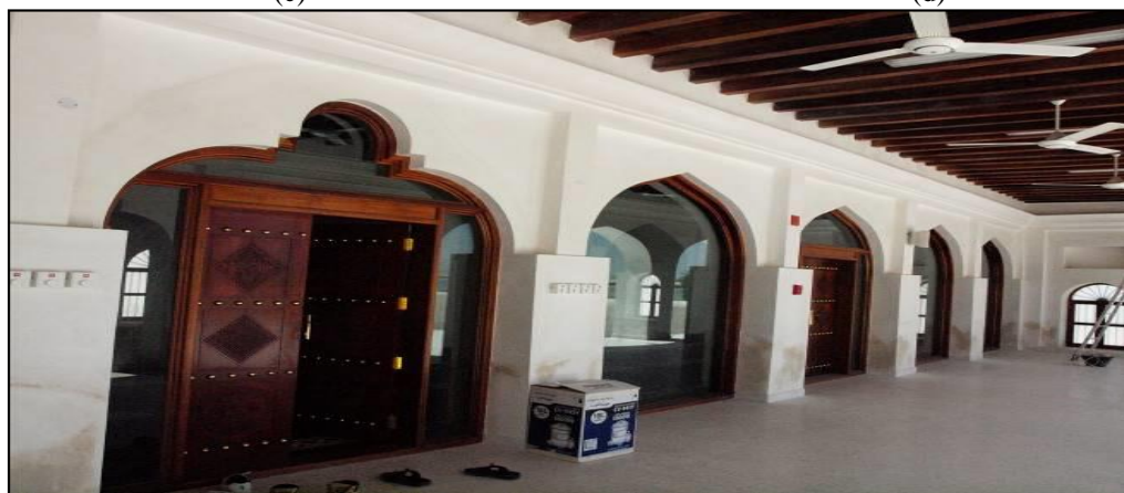
Figure 22. Mohammed ibn Abdul Wahab mosque in Al Thakhira, source: MEIA (a) Mosque floor plan, (b) Mosque elevations (c) the mosque before renovation, (d) the mosque after renovation (e) the entrance of the praying hall
