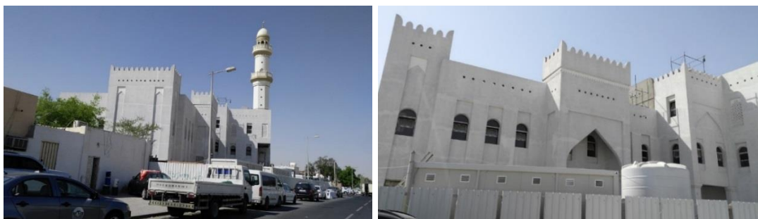
Figure 28. New mosque under construction at Al-Rayyan Al-Jadeed
