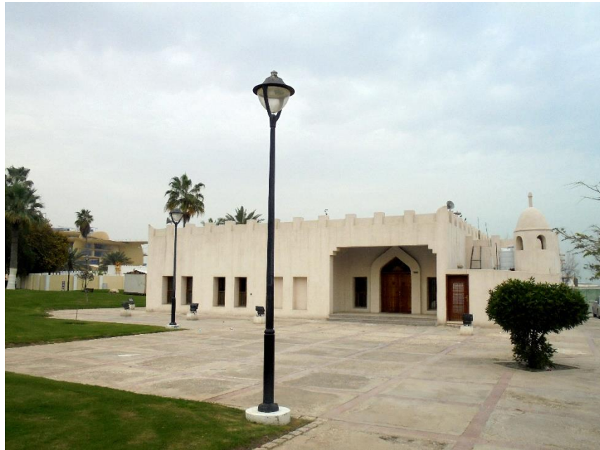
Figure 26. Ali bin Ali Al Khulaifi traditional mosque at Al-Cornish area, after renovation, source: the author
