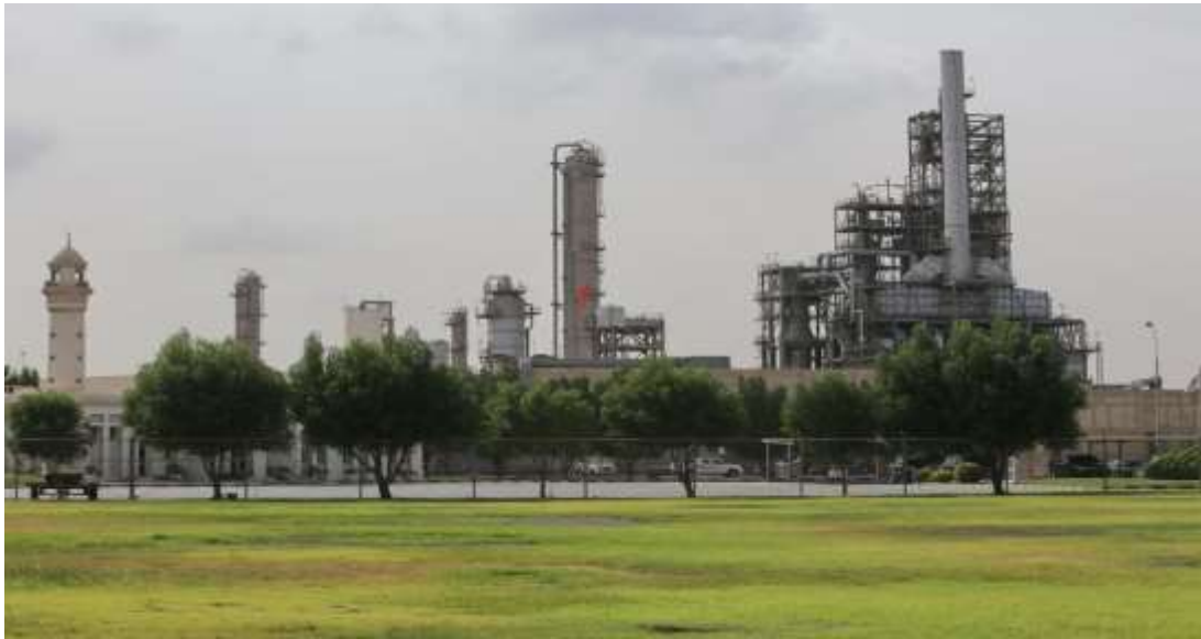
Figure 5. QAFAC plant in Mesaieed
