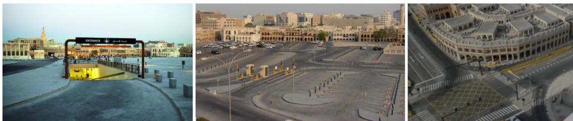
Figure 36. Parking provisions in the form of basement, above ground and MLCP (Source: Google earth, 2018)
