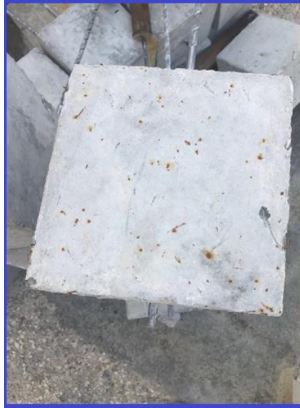
Figure 47: Corrosion of Steel Fibers in Steel FRC.
