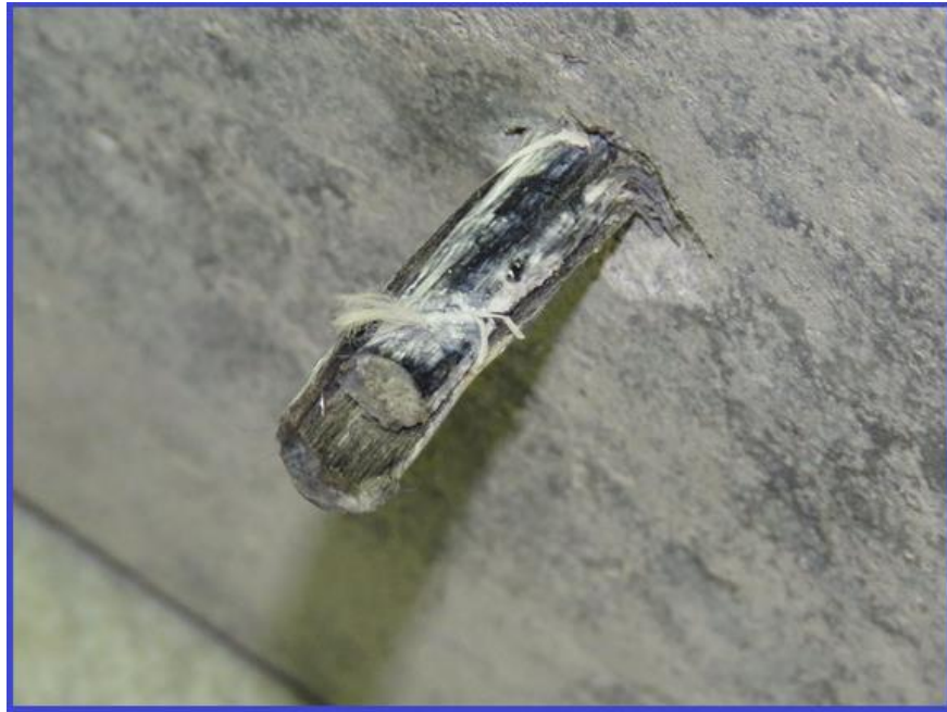
Figure 37: Complete Interlaminar Shear Failure between the Layers of the Bar.
