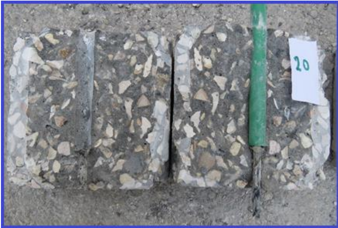
Figure 40: Closer Examination of conditioned Plain Concrete after 90 Days at 60 °C.
