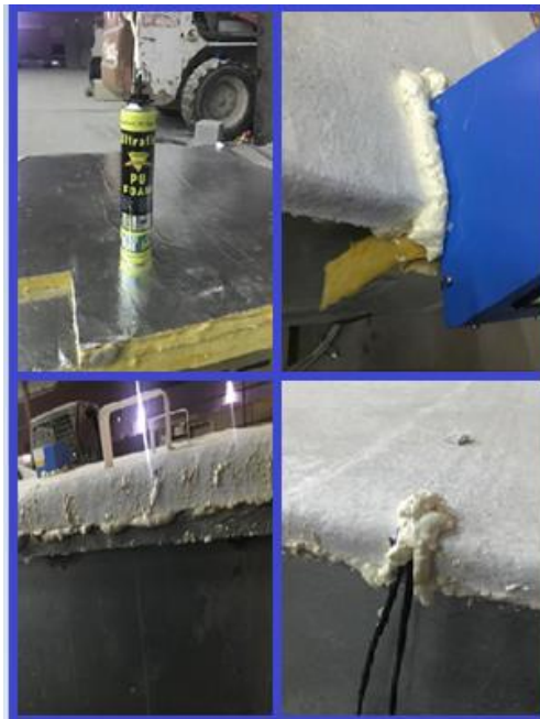
Figure 36: Polyfoam Used to Fill the Gaps and Openings.
