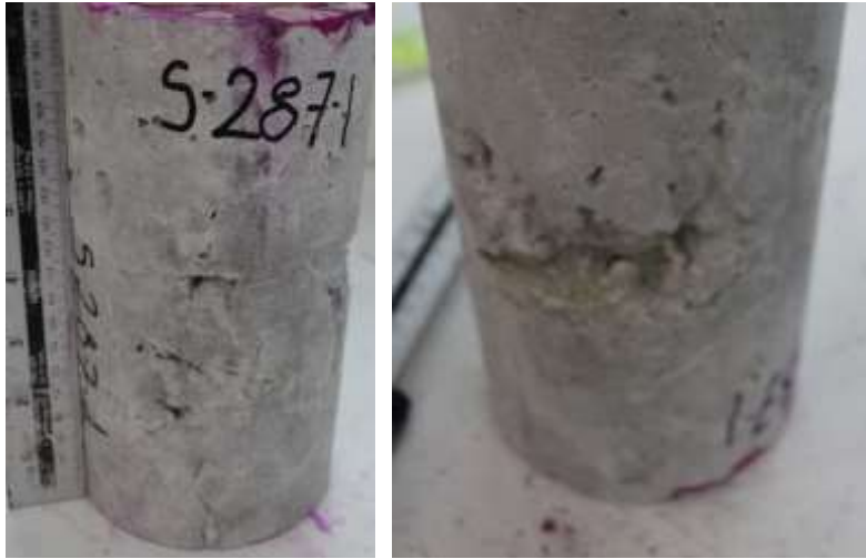
Figure 12: Voids and uncompact concrete in trial 1
