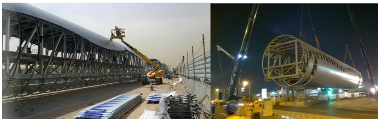
Figure 9: Off-site assembly and erection of typical span
