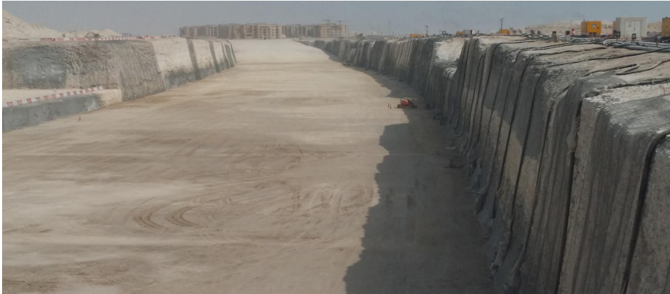
Figure 5: Completed excavation at the project site
