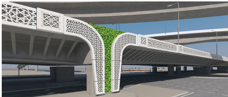
Figure 9: Arch Cladding at Select Piers of Sabah Al Ahmad Corridor.
