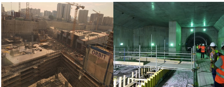
Figure 3: Overviews of construction condition during the planning stage
