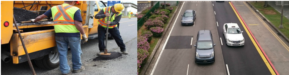
Figure 6: Prompt road maintenance on site
