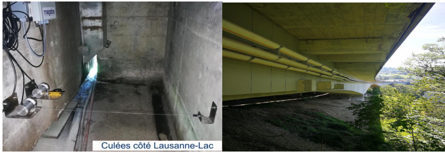
Figure 4: Lutrive River Bridge, Switzerland (left), and use of Lo-Ra wireless technology to transfer measured data from a sensor node to a gateway (right)
