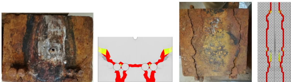
Figure 7: Crack pattern in a block specimen compared to previous FE results.
