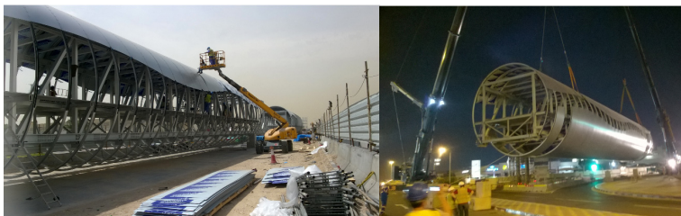
Figure 9: Off-site assembly and erection of typical span
