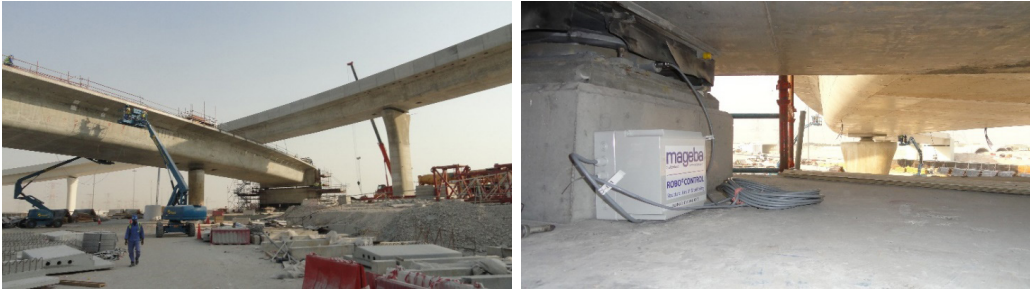
Figure 1: Construction of the main junction of the new Al Majd Road (formerly known as the Orbital Highway) in Qatar (left), and main sensor node of the project's SHM system, connected to bearings above (right)
