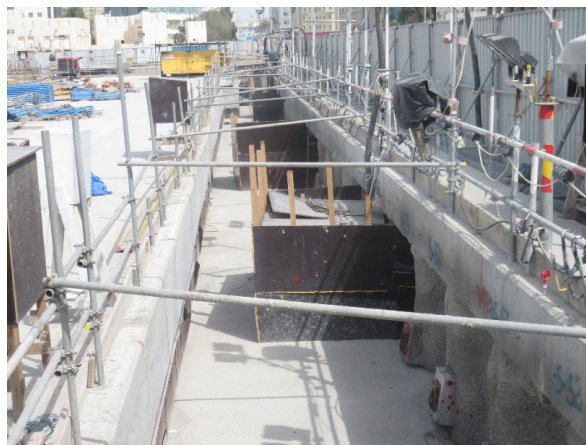
Figure 11: Encased dewatering well inside the lean concrete backfill
