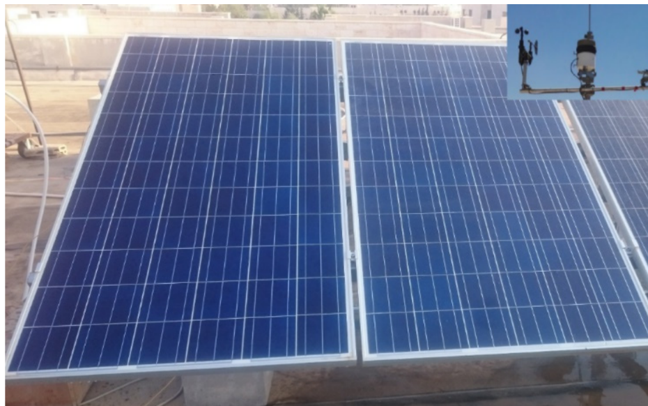
Figure 7. Solar Panels—YL300P-35P.
