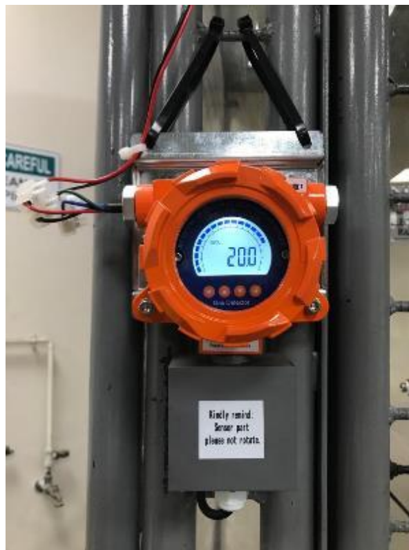
Figure 28. The OC-F08 gas detector
