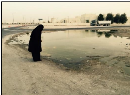
Leaking water from underneath some houses in Meaazer
