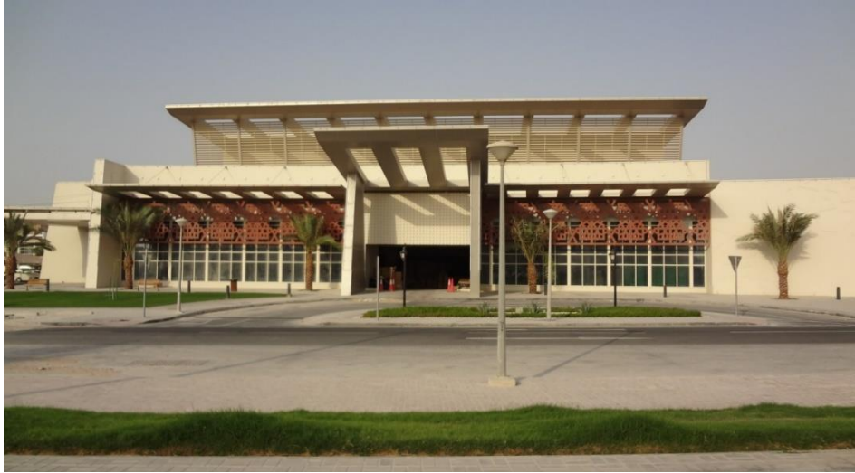
Figure 100: Shading Elements and Louvers on Building Façades: The Shopping Mall
