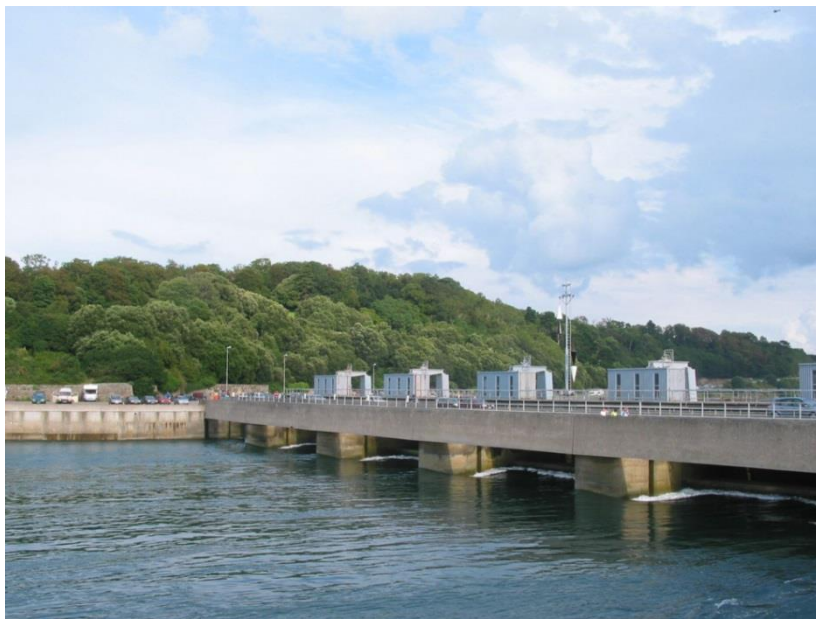
Figure 31: The Rance Tidal Power Station Bridges the Ranse River in Brittany, France (National Geographic, 2014)
