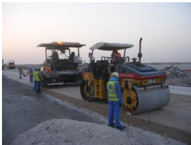
Figure 110: The First Road Made from Recycled Construction Materials in Qatar (Walker, 2015)
