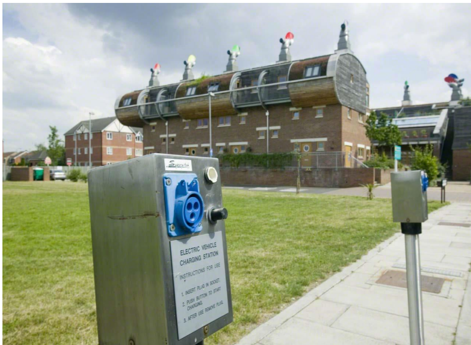
Figure 50: Electric Vehicle Charging Points at BedZED Powered by Renewable Energy, picture by (Ashley Cooper, 2007)
