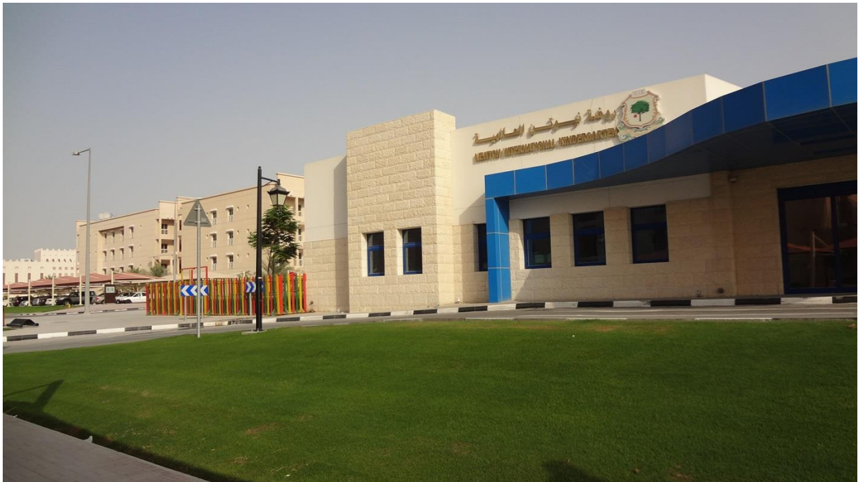
Figure 94: Newton Kindergarten in the Center of Barwa City
