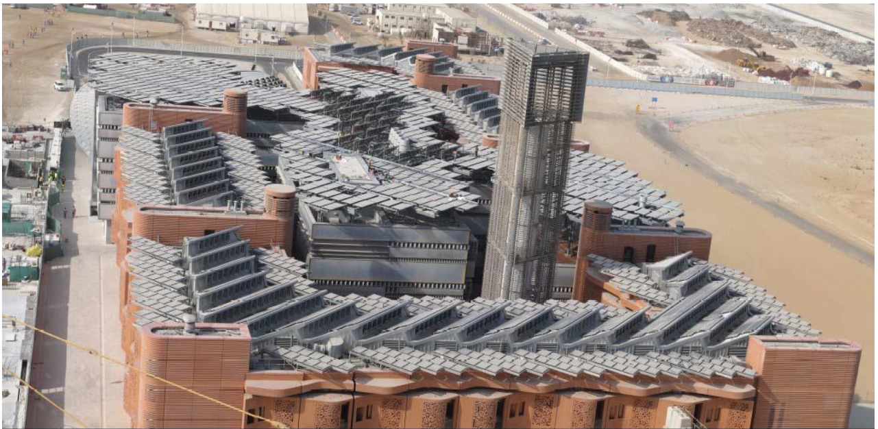
Figure 64: Rooftop Solar Panels Oriented to the Sun (Whittier, 2010)
