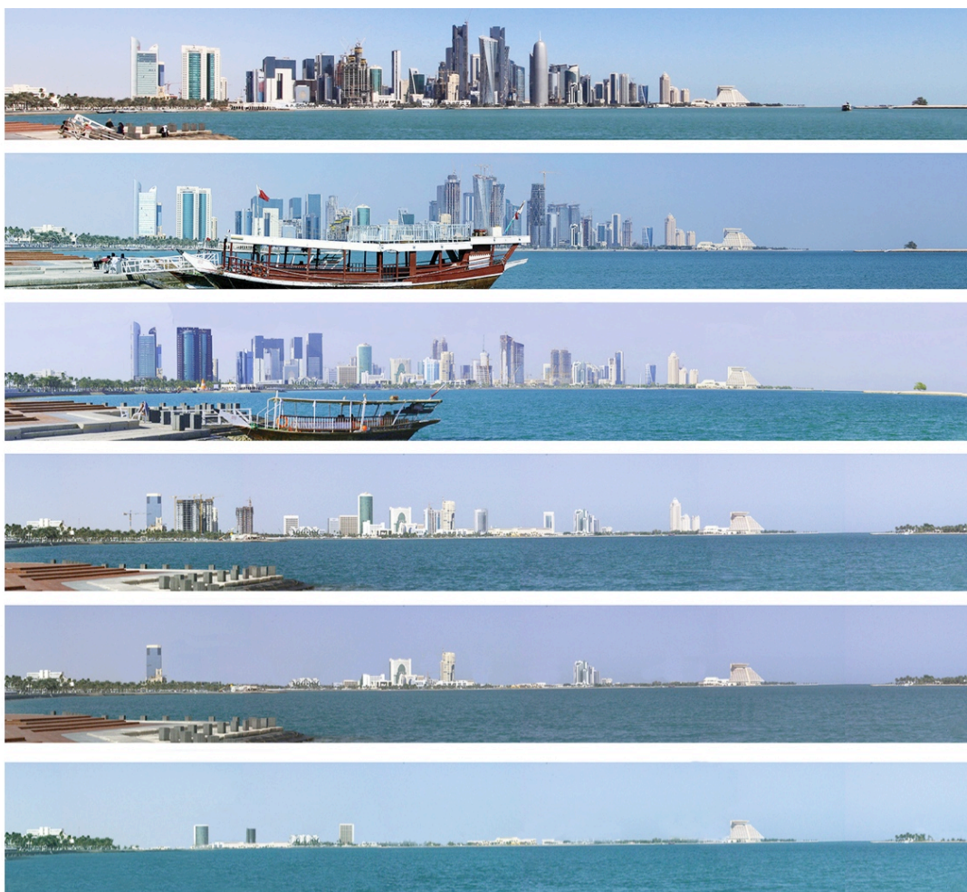
Figure 4.1. Doha skyline, 1985 to 2011, from bottom to top respectively.
