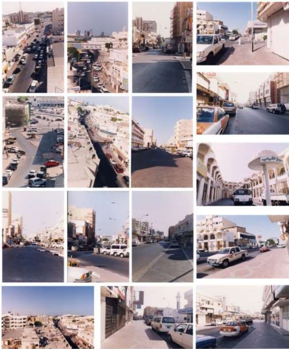
Figure 37 Kahrabaa Street in 2002, before the reconstruction, photos by the author
