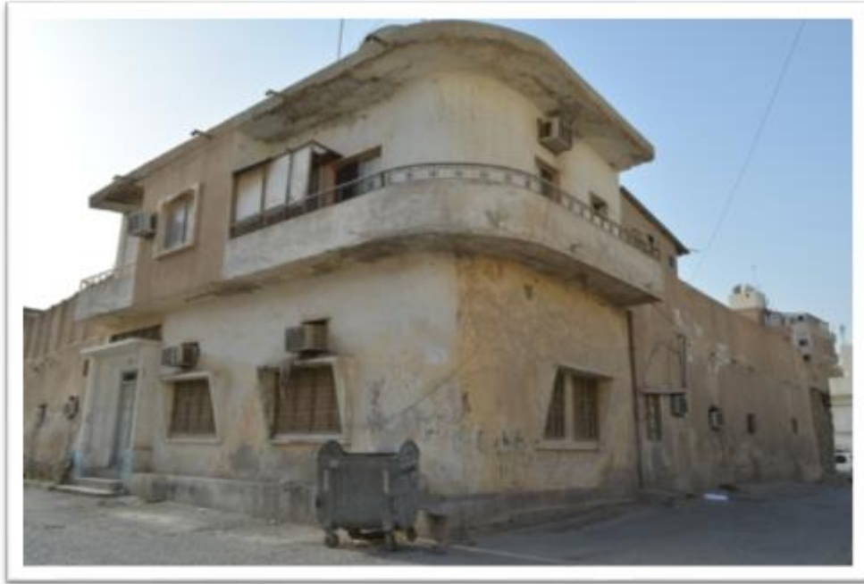
Figure 6-36. Amna Al Camal House Before Intervention
