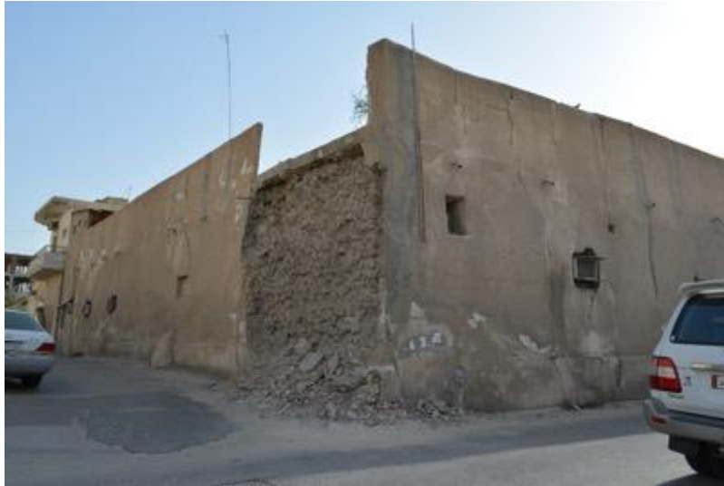
Figure 6-17. A Partly Demolished Wall (Source: Author)
