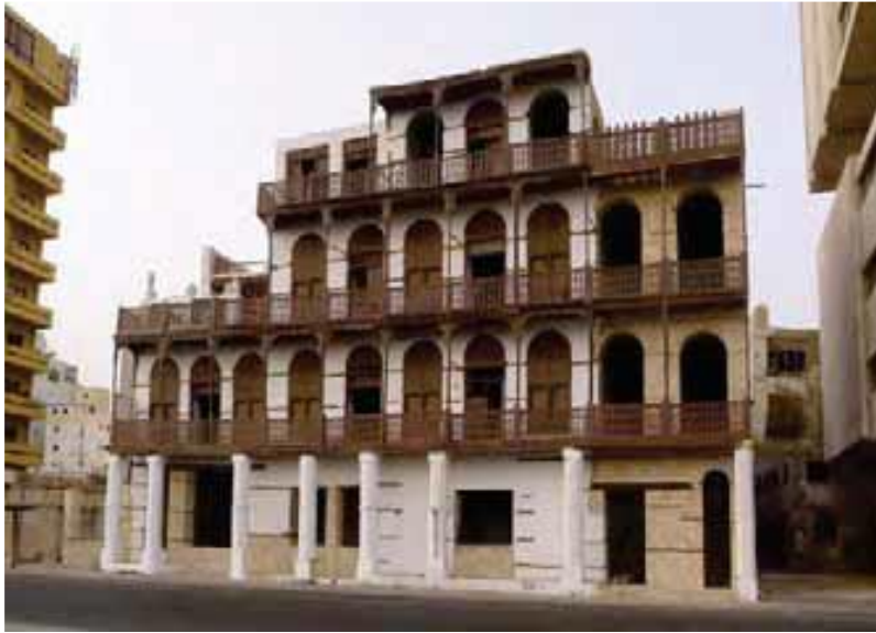
Figure 4-25. Jokhdar House (Source: Author)
