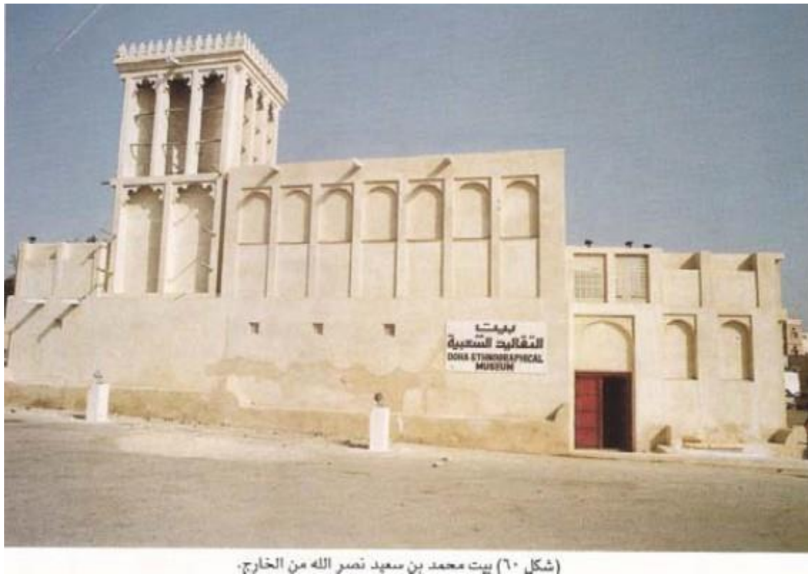
Figure 6-11. Mohammed Said Naserallah House (Source: QMA)
