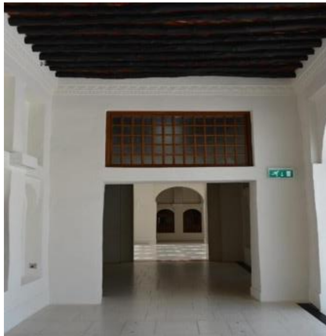
Figure 4-48. Roof structure (Source: Author)
