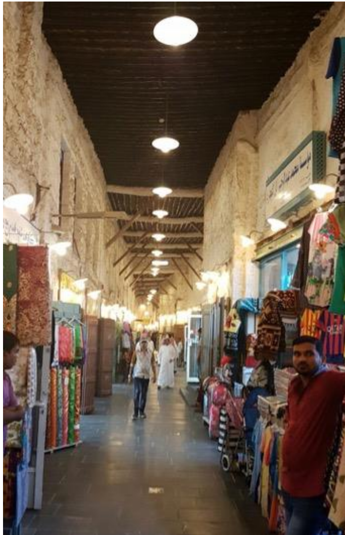
Figure 4-37. Bamboo Wood Roof System (Source: Author)
