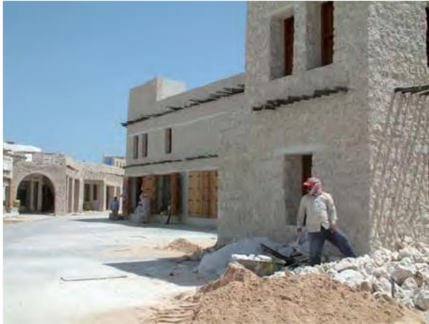
Figure 4-38. Restoration of Houses with Natural Stones Source: (Radoine, 2010)
