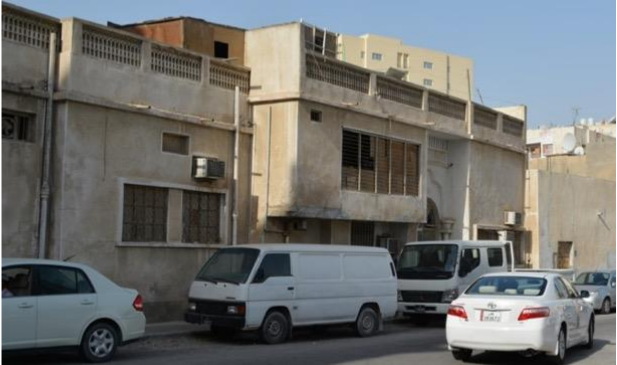
Figure 6-31. A View from Existing Buildings
