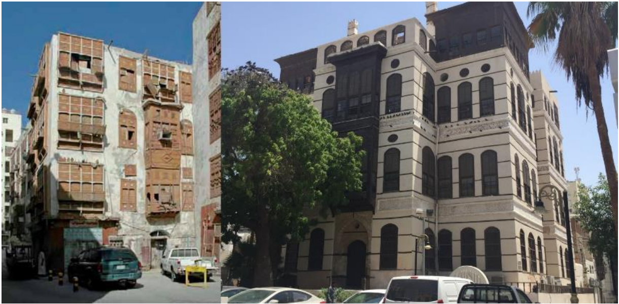
Figure 4-21. Before and After Rehabilitation of Naseef House (Source: Author)
