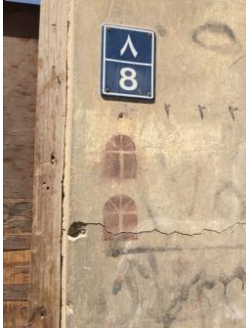
Figure 6-14. Marked Building (Source: QM)
