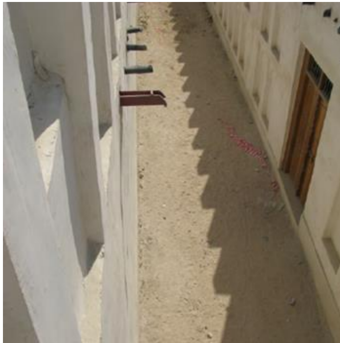
Figure 4-45. A view of a Sikkat (Source: (Msheireb: Heritage Quarter Houses Schematic Design Report, 2011)
