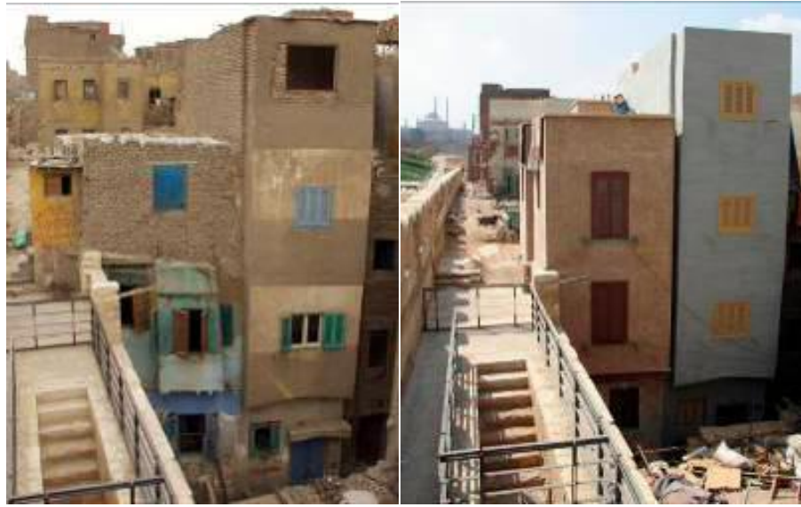
Figure 4-5. Before and After Rehabilitation (Khasaba, 2011, p. 2)
