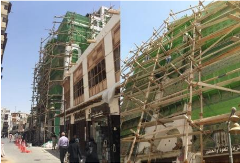
Figure 4-22. Restoration of Noorwali House (Source: Author)
