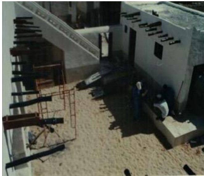
Figure 6-13. Building Number 10 During Restoration Work (Source QM)
