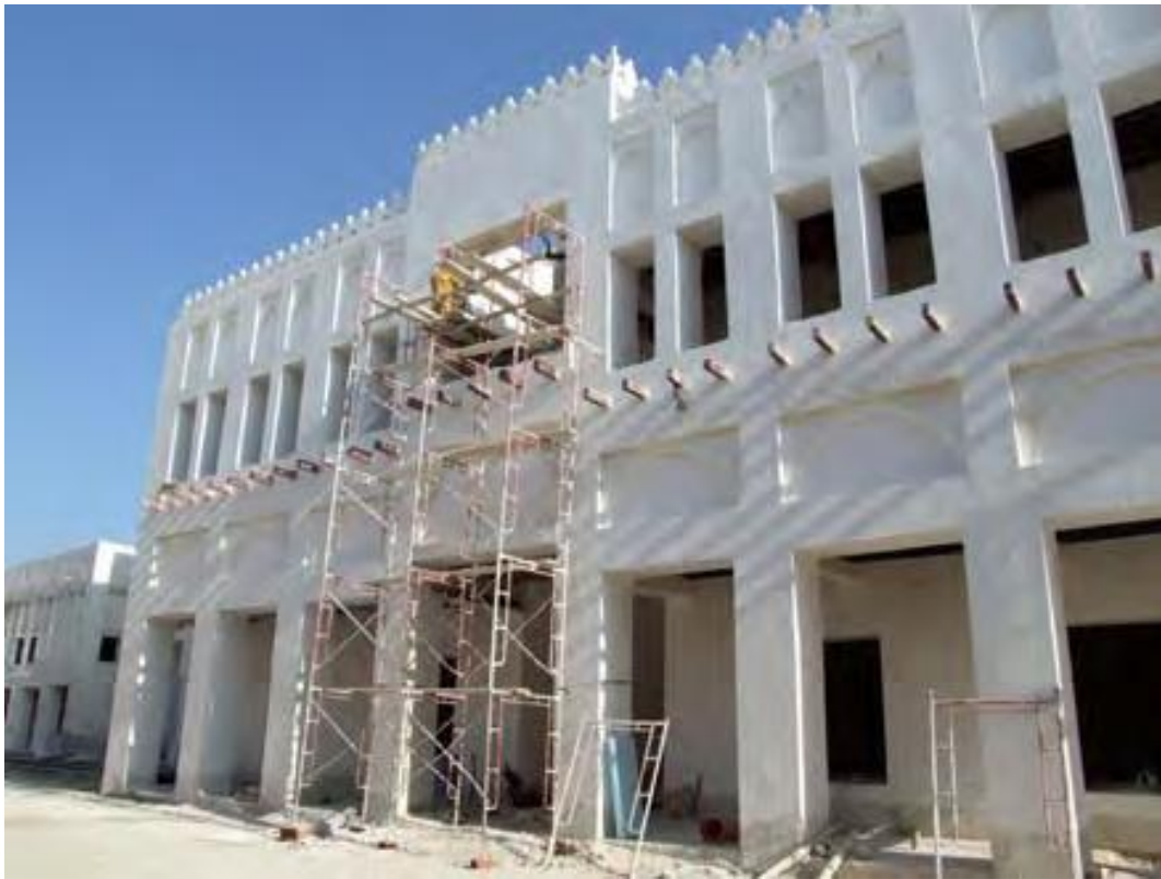
Figure 4-35. Restoration of Building in Souq Waqif (Radoine, 2010)
