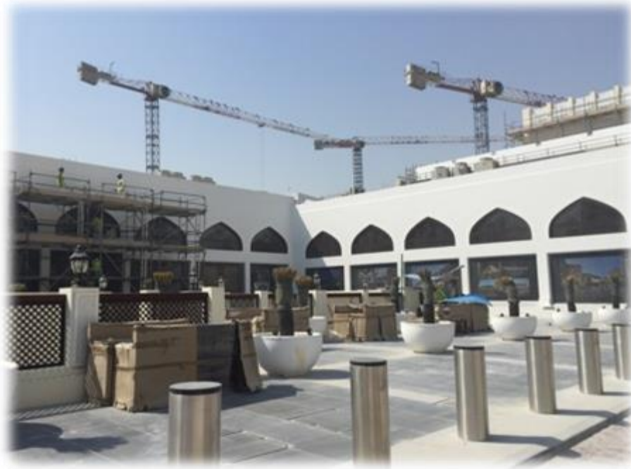
Figure 6-27. New Mixed Use Complex
