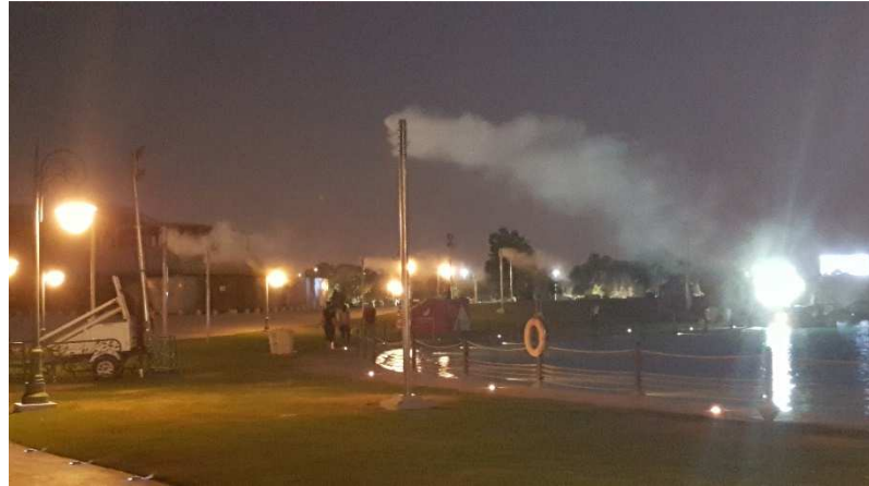
Figure 66. Evaporative cooling device in Aspire (source: author)
