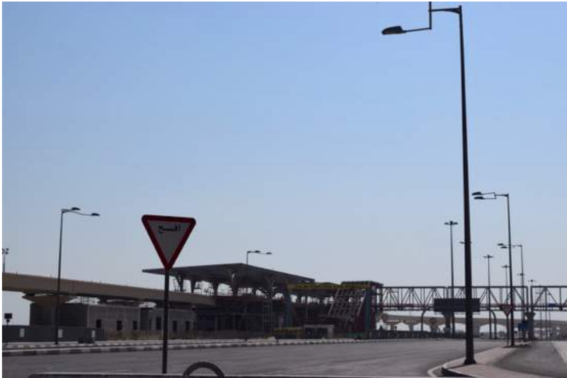
Figure 120. The under construction Al Wakrah metro stop on the red line.
