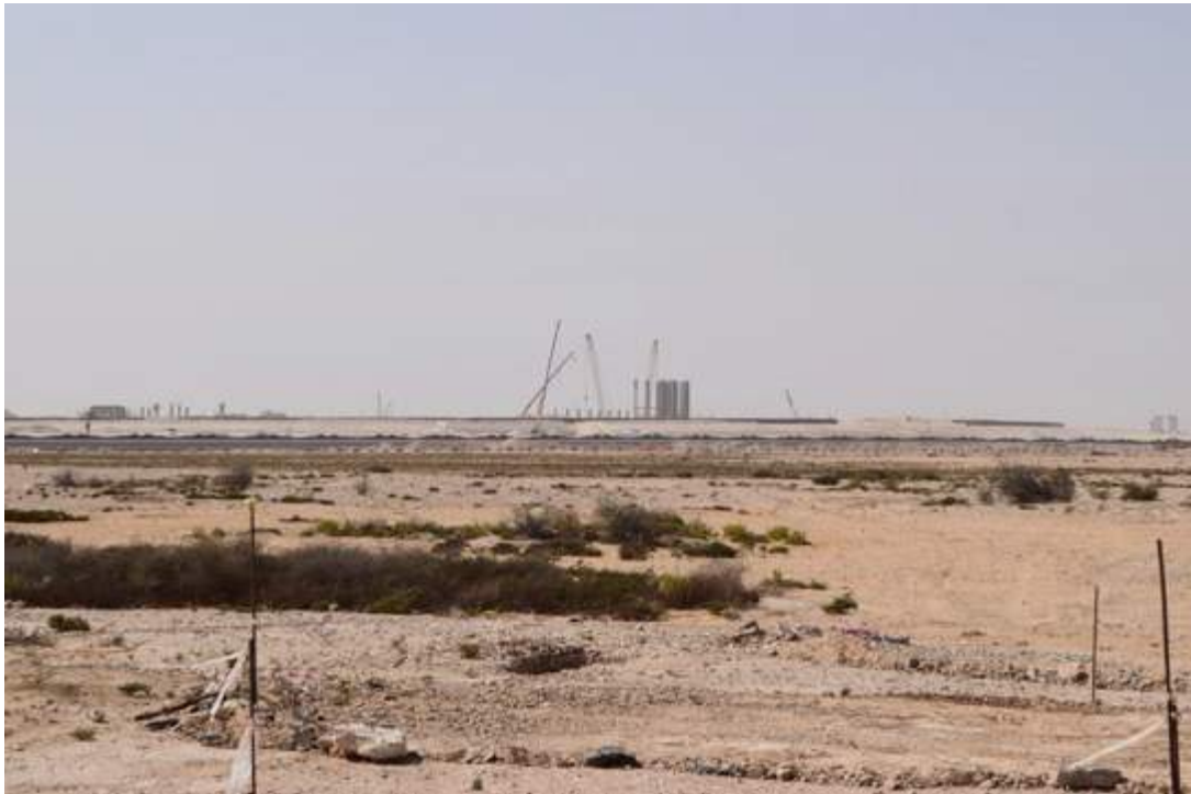
Figure 114. Works at Al Khor stadium.
