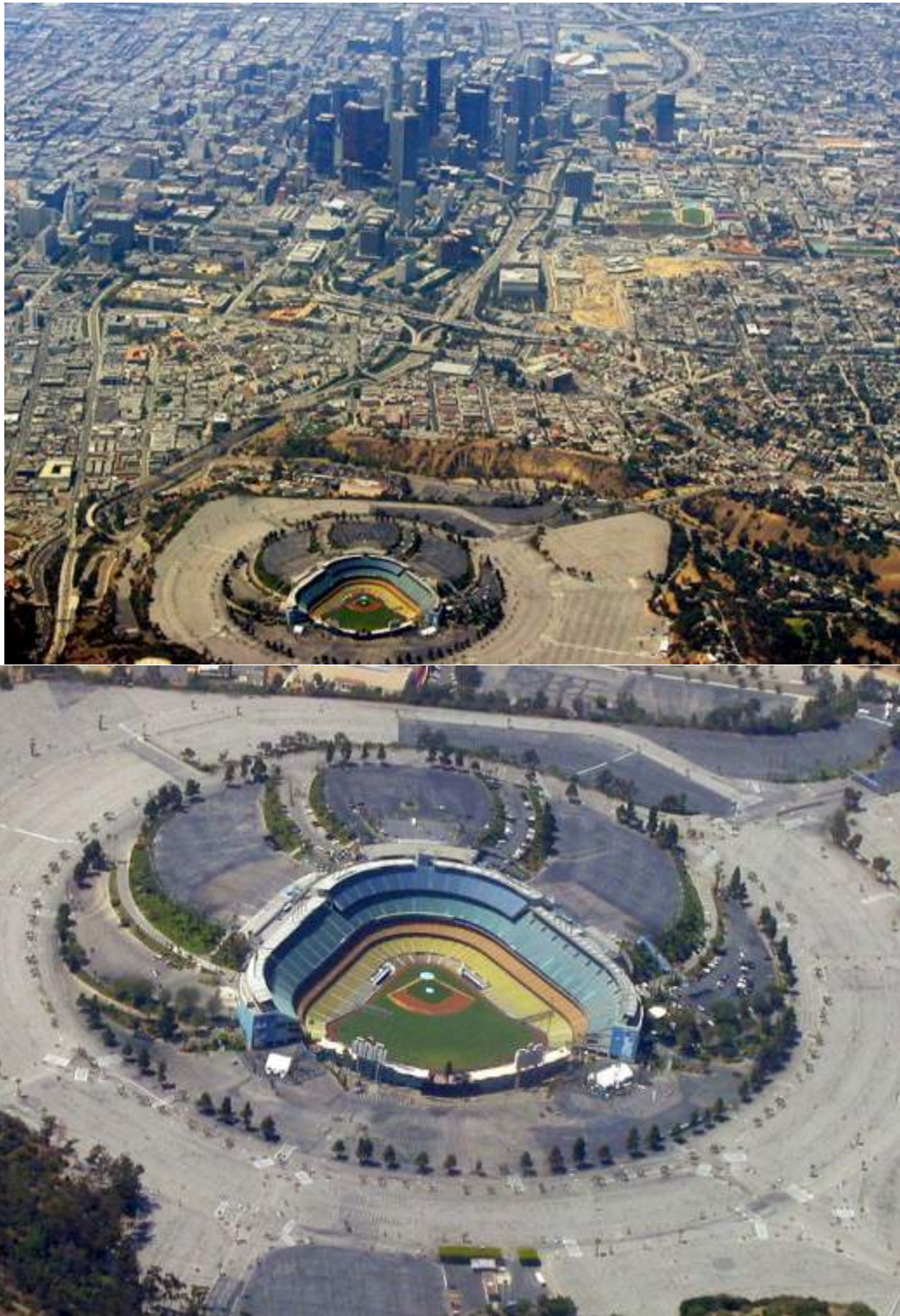
Figure 36. Dodgers Stadium in Los Angeles, a gigantic 'hole' within the urban fabric (Source: Ron Reiring, under the Creative Commons Attribution 2.0 Generic license).
