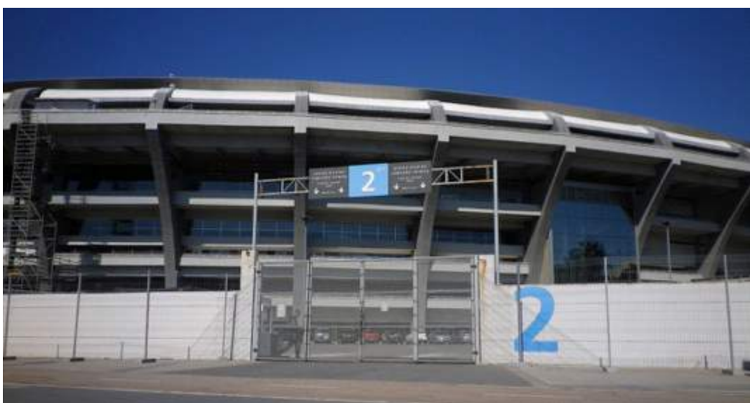
Figure 92. One of the gates to Maracanã stadium.
