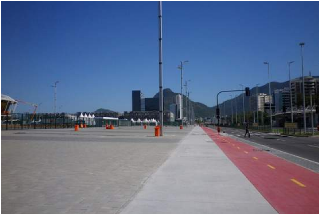
Figure 85. The cycling path around the Olympic Park.
