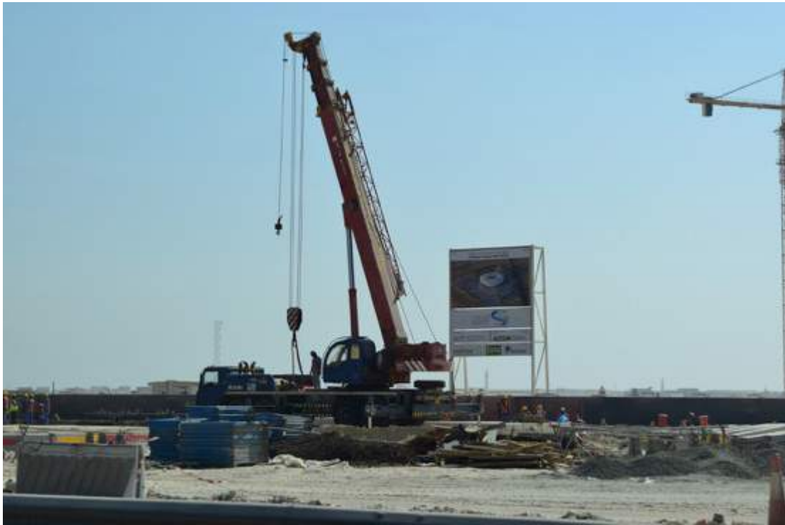
Figure 123. Works at the stadium.
