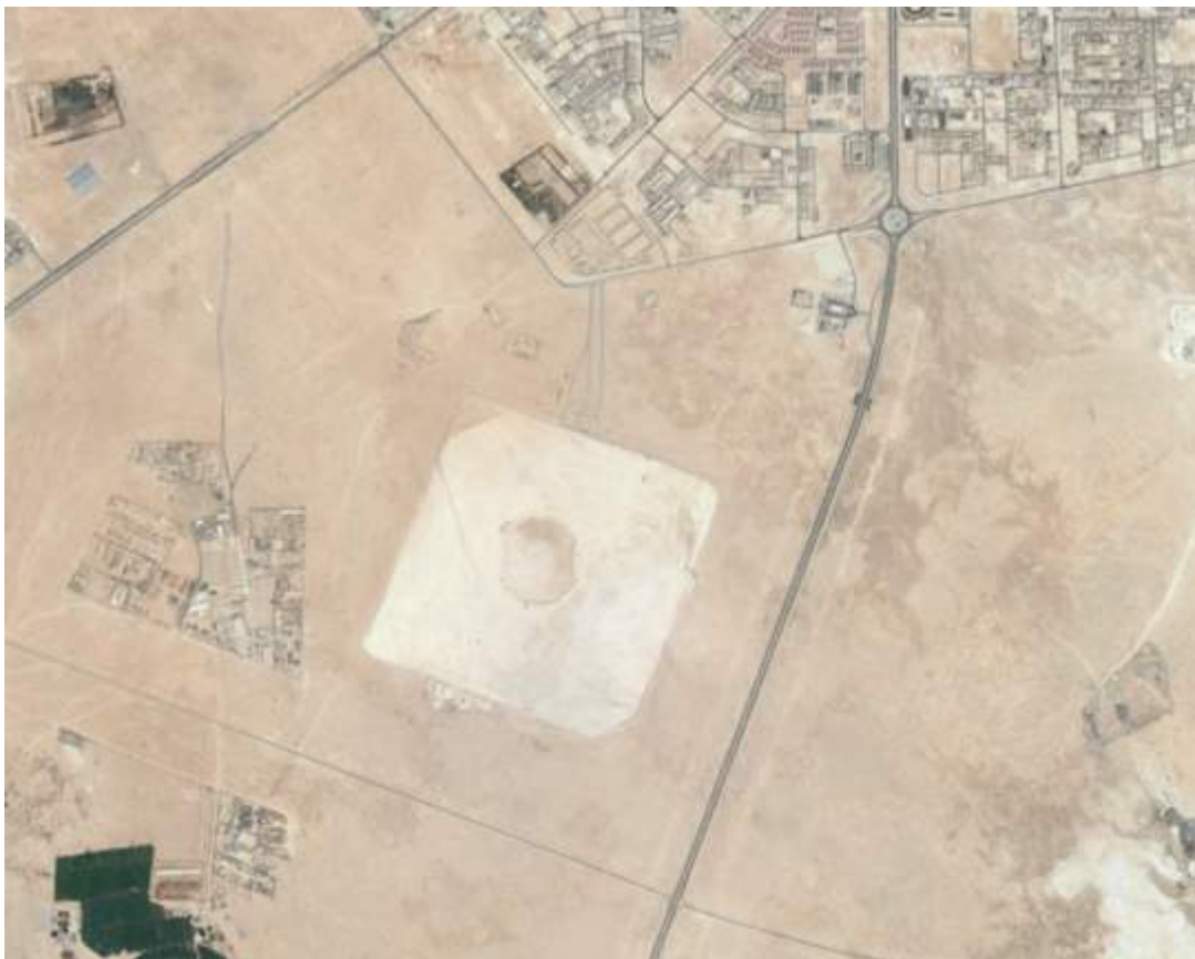
Figure 115. Aerial view of Al Khor stadium (Adapted from Google Earth).
