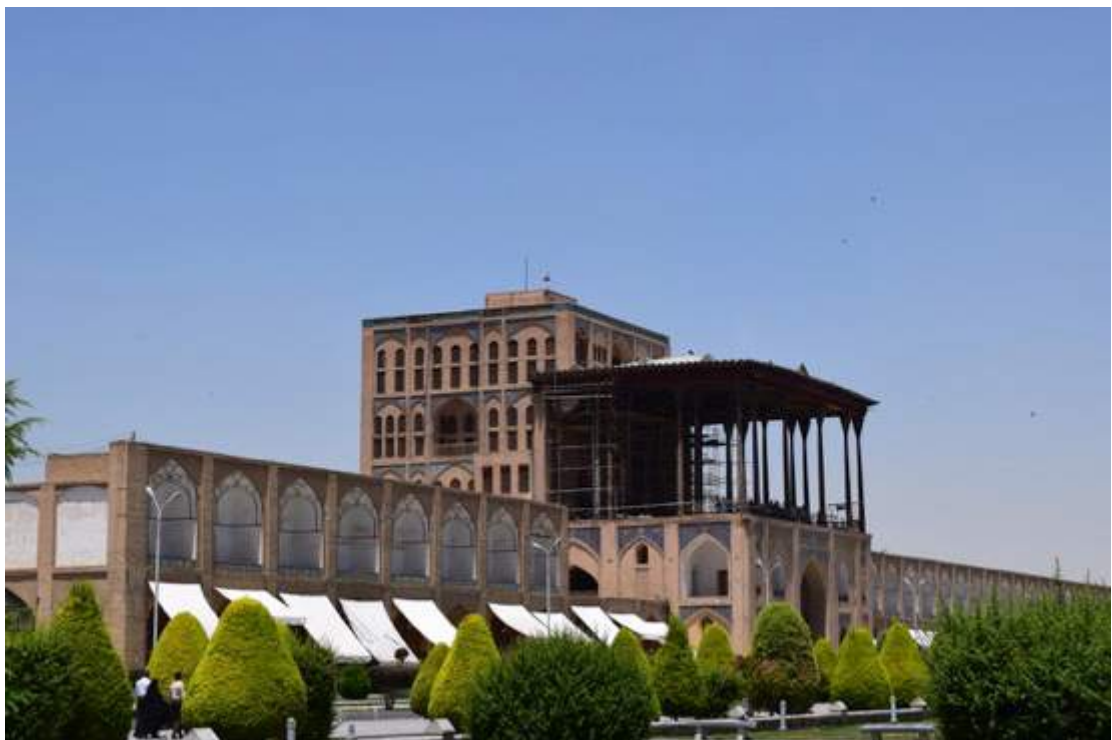
Figure 30. Esfahan, the Royal palace with the terrace facing the square (Source: Author).
