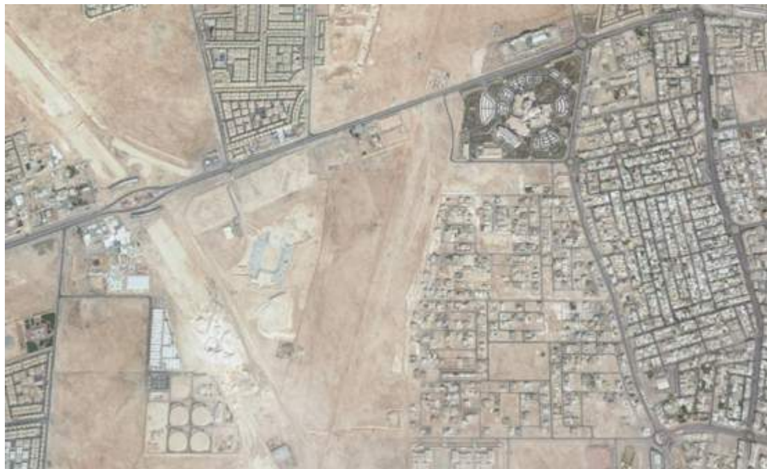
Figure 122. Aerial view of Al Wakrah stadium.
