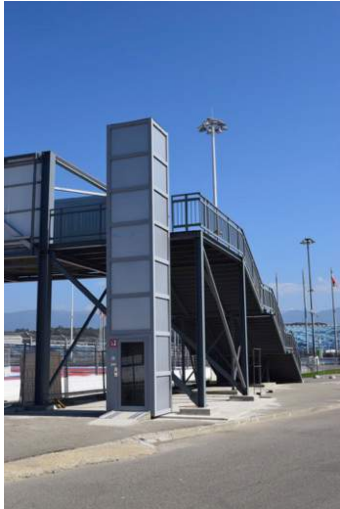
Figure 70. A detail of the bridge that overpasses the F1 track and cuts the Olympic Park.
