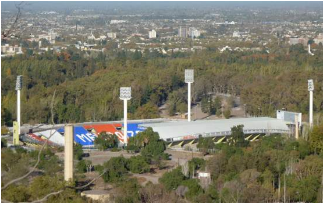
Figure 38. Stadium in Mendoza, Argentina (Source: Dr. Haus, under the Creative Commons Attribution-Share Alike 3.0 Unported license). The stadium, built for the 1978 World Cup, was planned to disguise itself in the surrounding landscape. It is partially underground (De Ambrosis, 2013).
