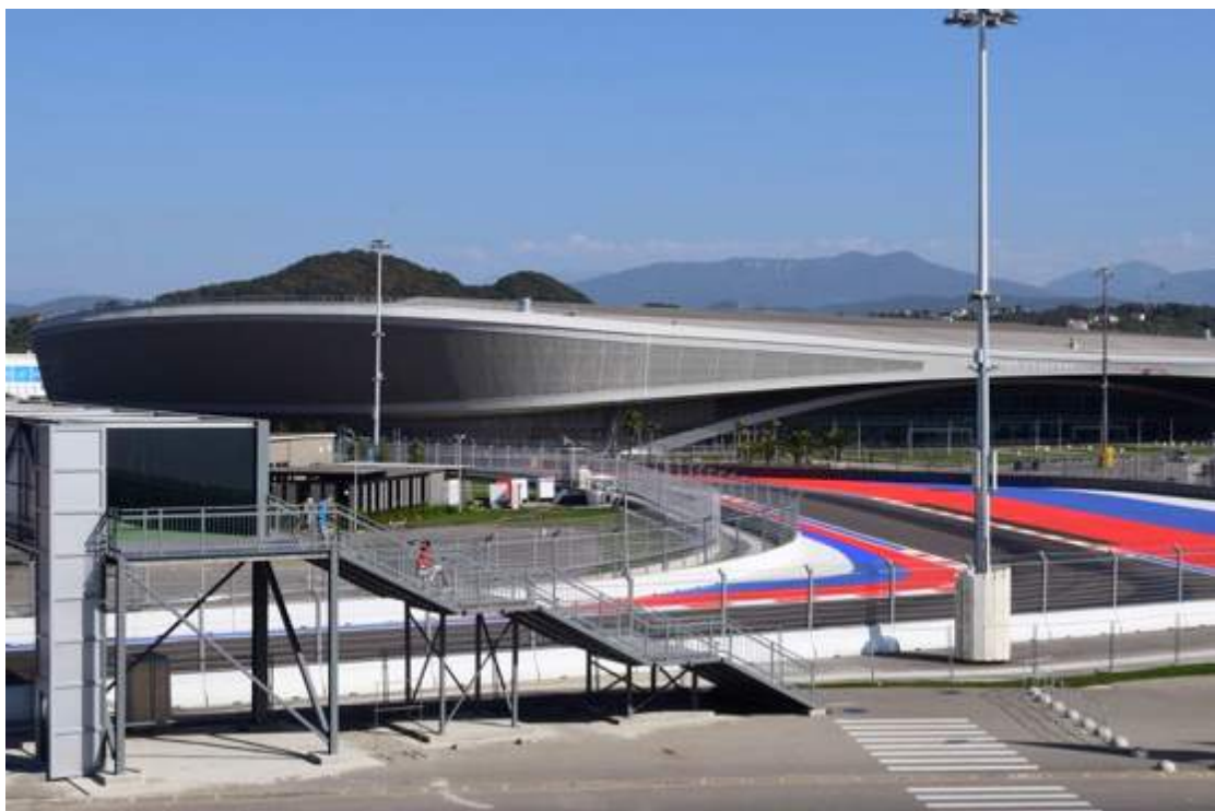
Figure 69. One of the four bridges that overpasses the F1 track and cuts the Olympic Park.
