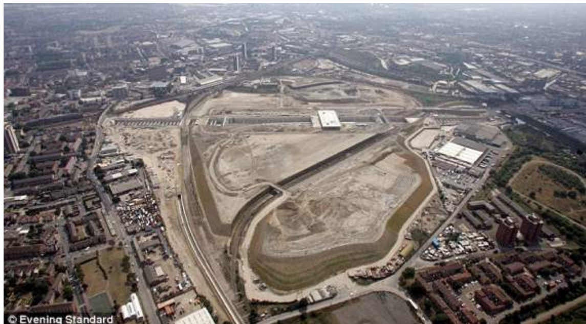
Figure 46. London Olympic Park before the regeneration project for the Games. Source: Daily Mail.
