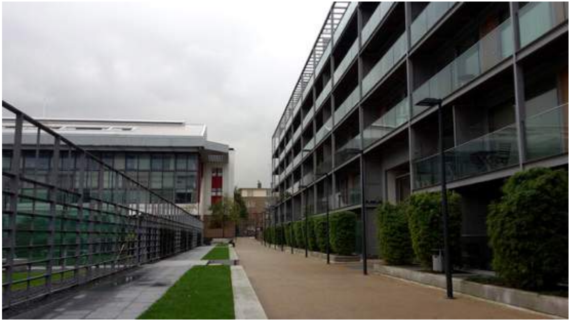
Figure 135. The former Arsenal stadium, now Highbury Square, a complex of about 700 apartments.
