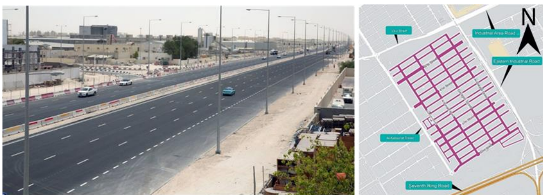
Figure 11. The work on the third package of the streets and infrastructure project in the Doha Industrial Area has been completed—source (Ashghal,2024).
