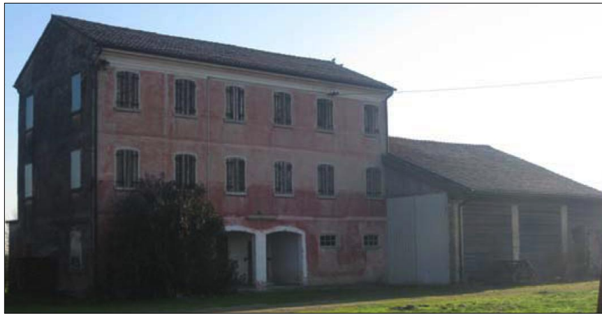
Figure 1. Extended Family House in Italy
