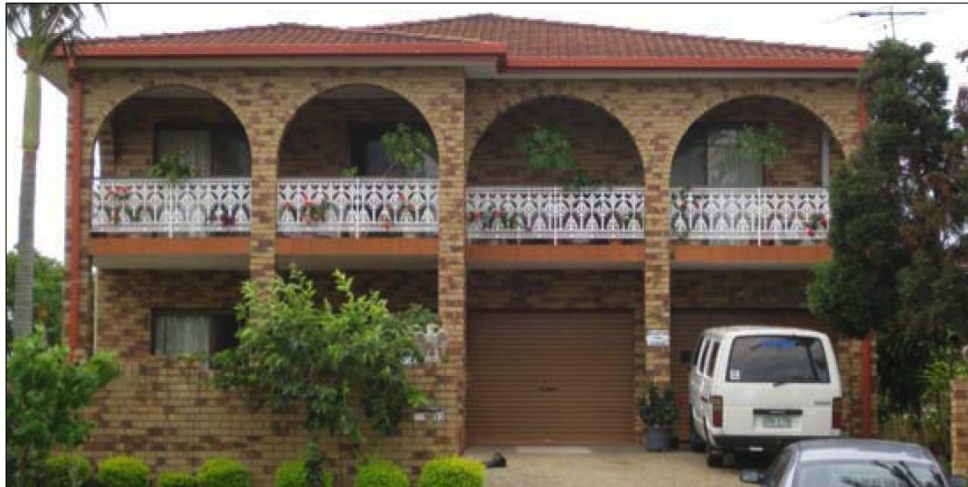
Figure 8. Front façade of Italo-Australian house (case 2)
