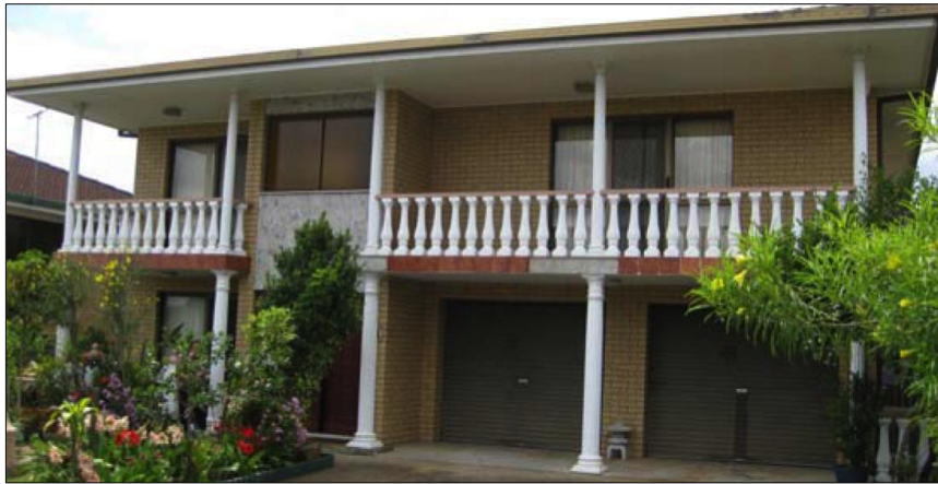
Figure 5. Front façade of Italo-Australian house (case 1)
