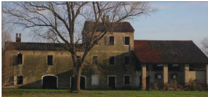
Figure 2. Extended Family House in Italy
