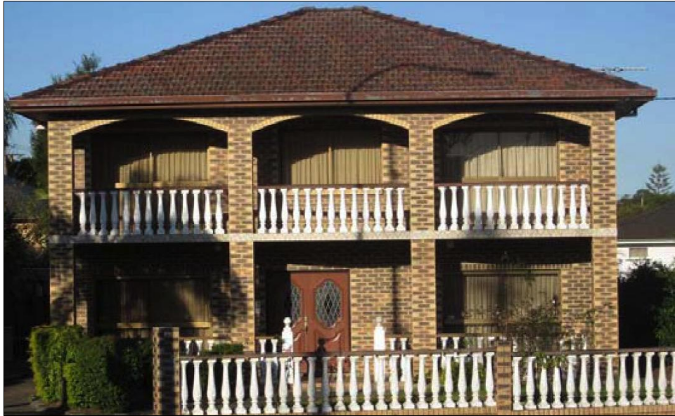
Figure 14. Front faade of Italo-Australian house (case 4)
