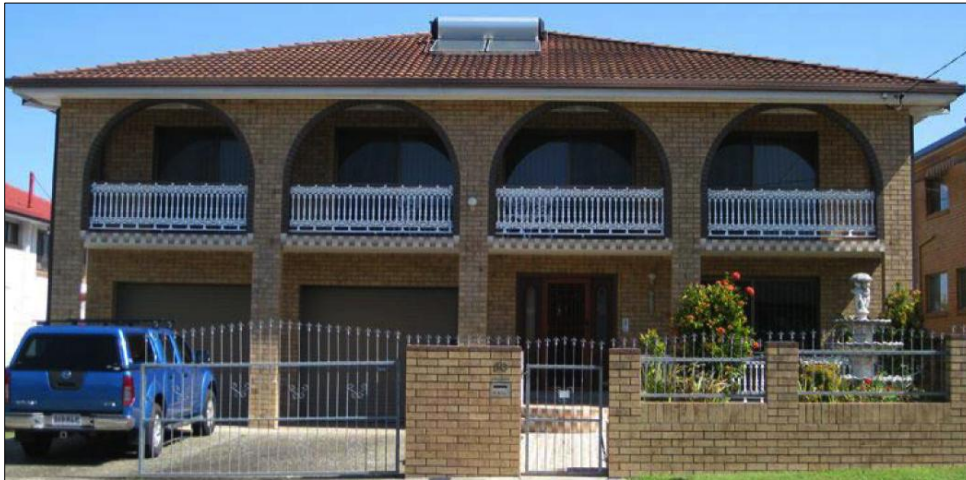
Figure 11. Front façade of Italo-Australian house (case 3)
