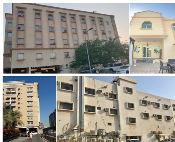
Fig. 1. Typical buildings surveyed
