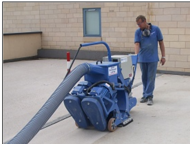
Figure 4: Shot blasting equipment [37]
