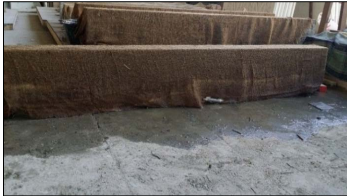
Figure 20: Saturating the beam specimens prior of strengthening
