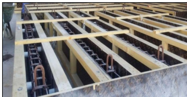
Figure 16: Steel reinforcement cages inside the wooden form work
