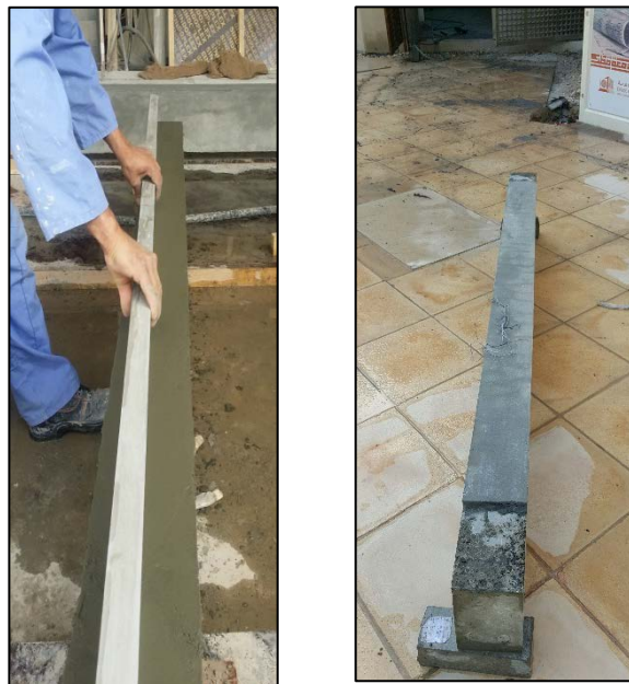
Figure 25: Final layer of mortar laying and finishing
