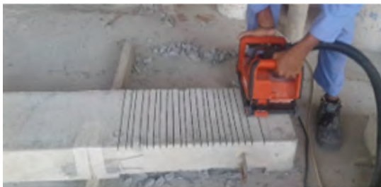
a) Cutting groove with slitting machine.
