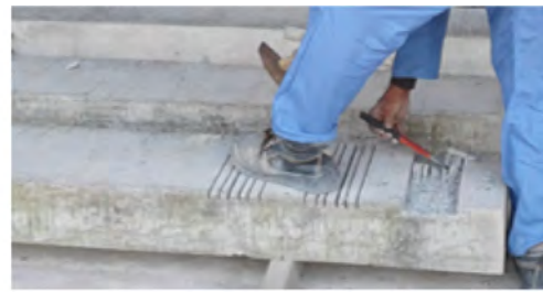
b) Removal of concrete between the grooves.
