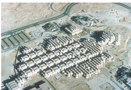
FIGURE 3: Aerial view of Qatar University campus: early stages of implementation.
