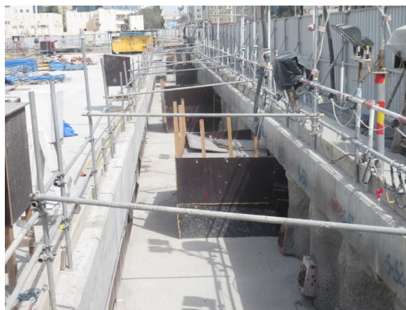
Figure 11: Encased dewatering well inside the lean concrete backfill
