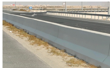
(b) Concrete barrier (rigid)
