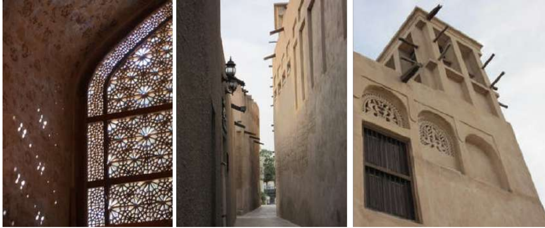
Figure 21: (left) Lattice windows, (center) Narrow streets Built close, for comfort, and (right) a wind tower (Source: Felibrilu/Flickr, CC BY-NC).
