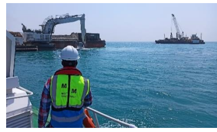
Backfilling in process
