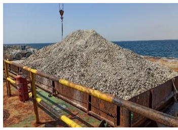
Reused back filling material
