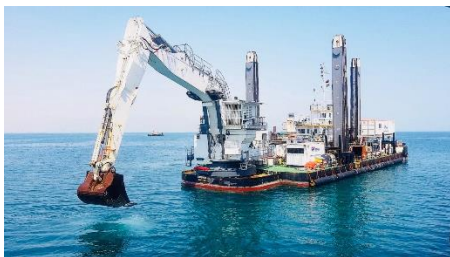
Backfilling barge and excavator
