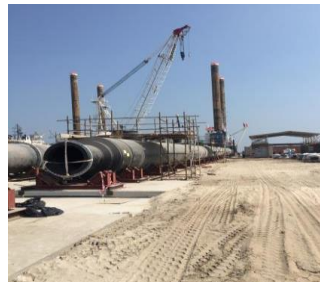
HDPE pipework being assembled
