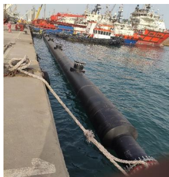
Pipe section ready for towing
