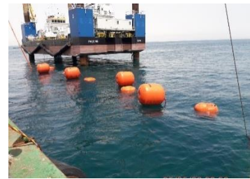
Submerging the pipe
