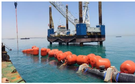
Pipe section with buoyancy aids
